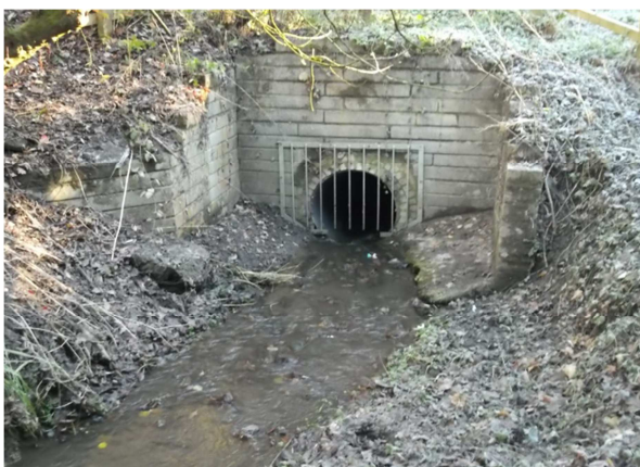
3. Culvert Inlet – Rhos_0362 ESTRY Unit: Circular Culvert
