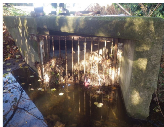
2. Culvert Inlet – Rhos_1059 ESTRY Unit: Circular Culvert
