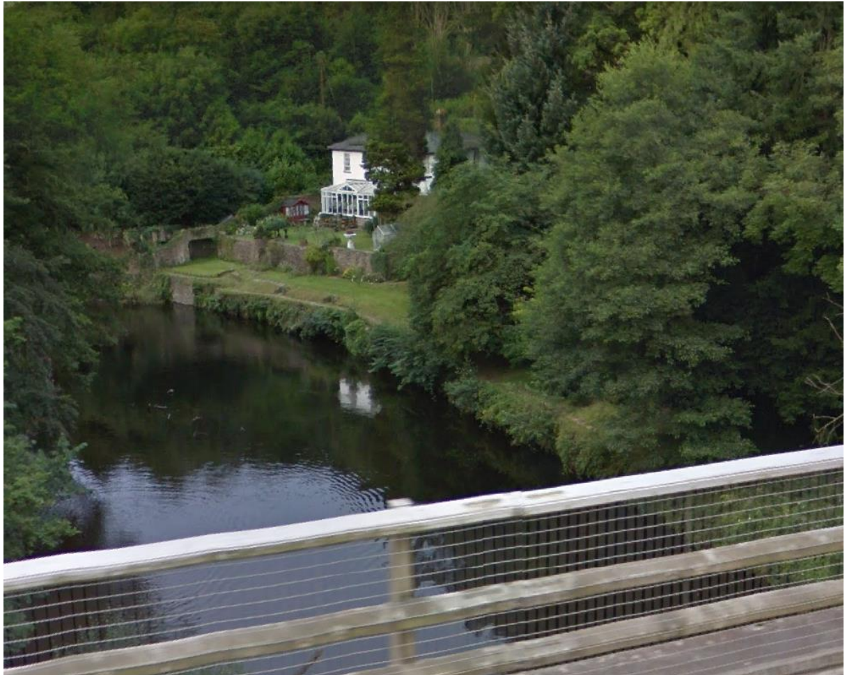
Figure 5. Existing Extension at Dee House
