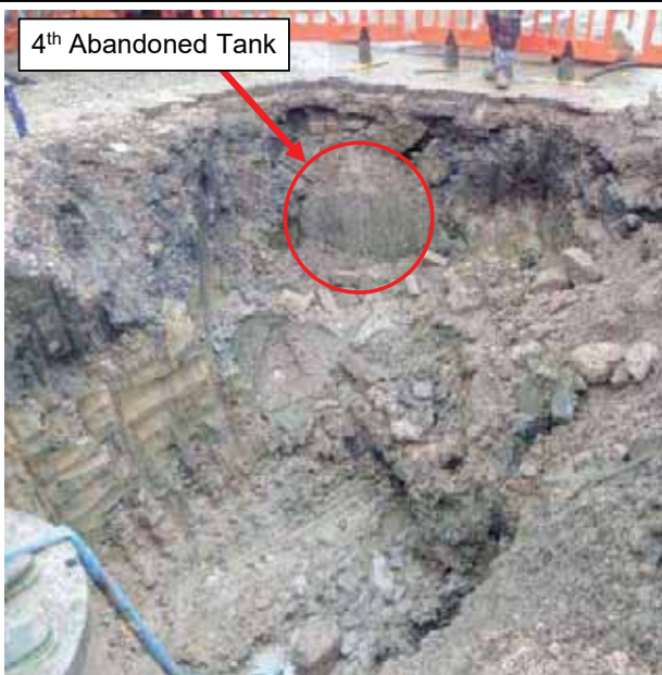
Photograph Twenty-Eight - EX201 following removal of third abandoned tank. Fourth abandoned tank visible in northern wall of the excavation.
