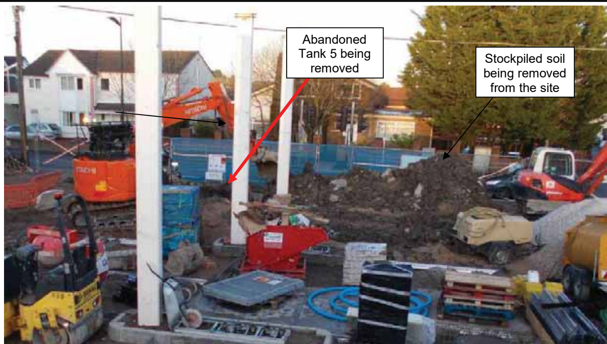
Photograph Thirty-Two - Overlooking construction site towards fifth abandoned tank
