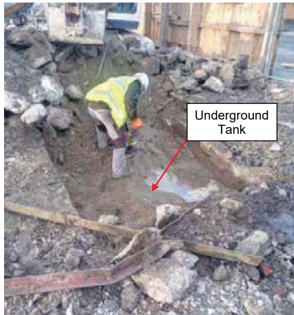
Photograph Fifteen - Exposing abandoned tank at the front of the site.
