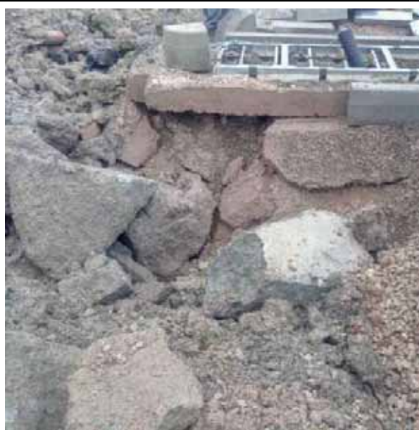
Photograph Twenty-One - EX301, excavation extended to allow delineation of the observed possible hydrocarbon impact.
