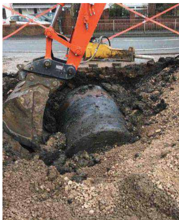
Photograph Thirty-One - Abandoned tank being removed
