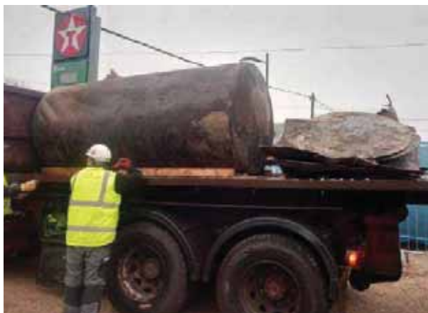
Photograph Eighteen - Abandoned tanks removed from the site.
