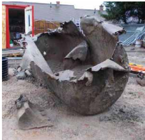
Photograph Twenty-Seven- Abandoned tank #3 after it had been removed
