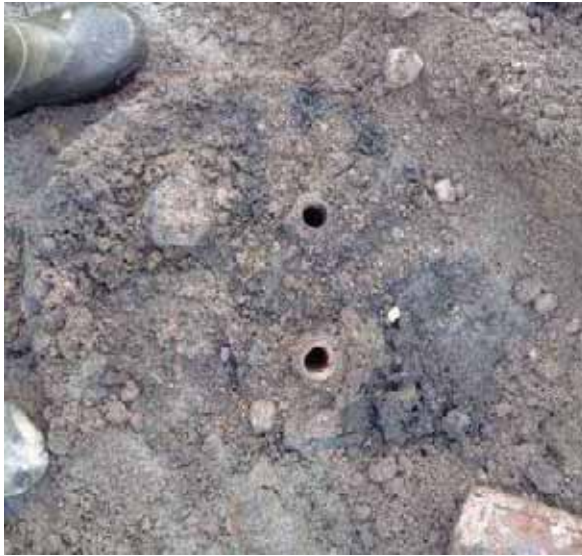
Photograph Sixteen - Lid of abandoned tank with fill point and vent holes visible.
