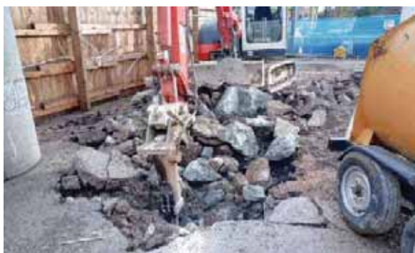
Photograph Eleven - Breaking ground at front of site
