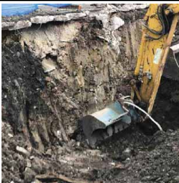
Photograph Nine - Digging to base of tank depth in EX001 (note clean clay soils)
