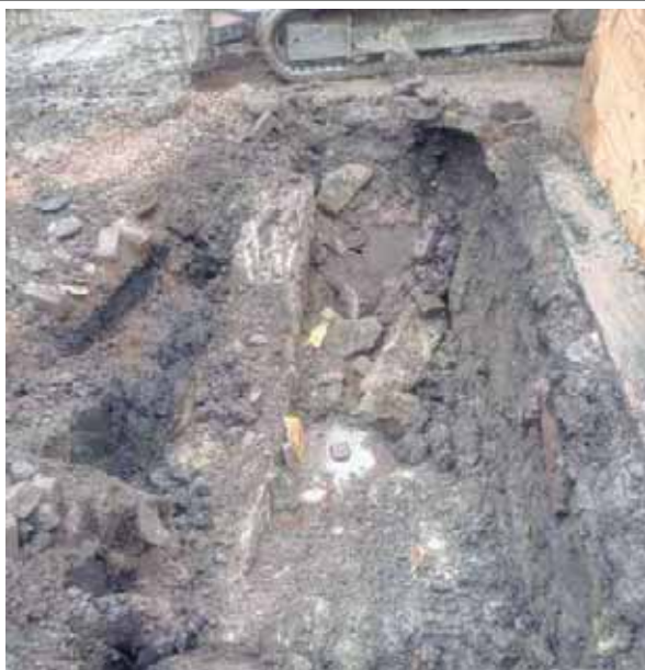
Photograph Twenty-Four - Interceptor being removed. Large concrete cradle on eastern wall. Impacted soil beyond cradle
