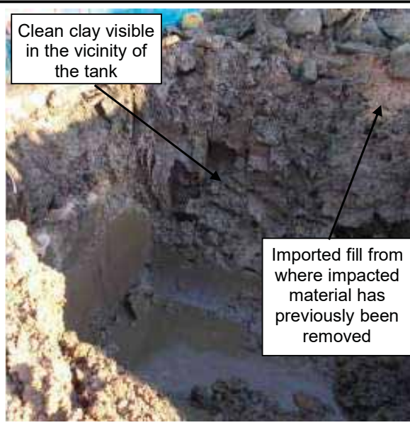
Photograph Thirty-Seven - Clean clay visible on the excavation walls - imported fill from previous impacted soil removal visible
