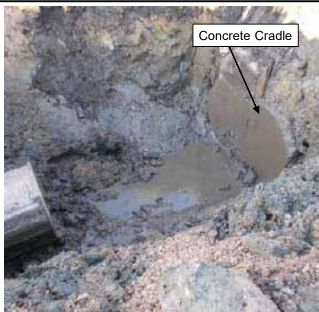
Photograph Thirty-Six - Concrete cradle remaining after Abandoned Tank 5 has been removed
