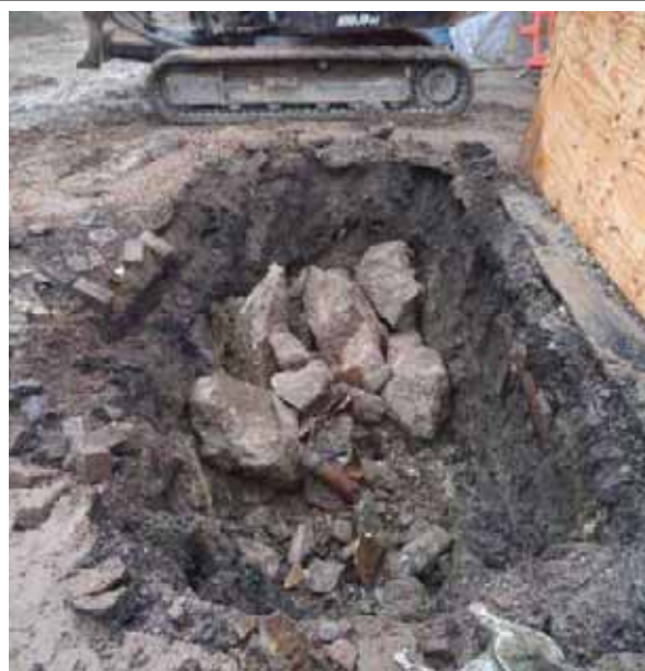
Photograph Twenty-Five - Interceptor and concrete cradle removed.
