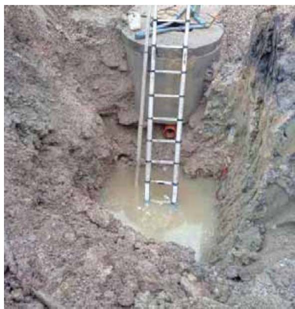
Photograph Twenty-Nine - EX201, excavation prepared for interceptor installation. Water pooling at the base of the excavation.
