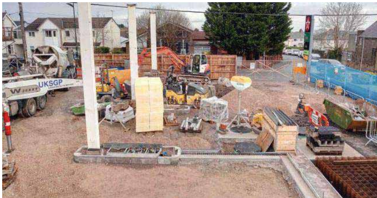
Photograph Thirteen - Site overview: Excavator at front of site breaking out concrete
