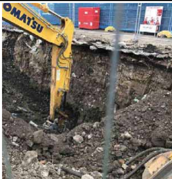
Photograph Ten - Digging to the base of the tank farm in EX001
