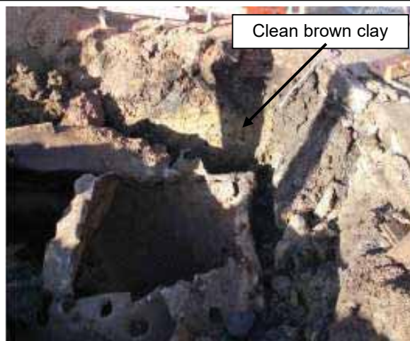
Photograph Thirty-Five - Visible brown "Clean" Clay exposed around abandoned Tank 5
