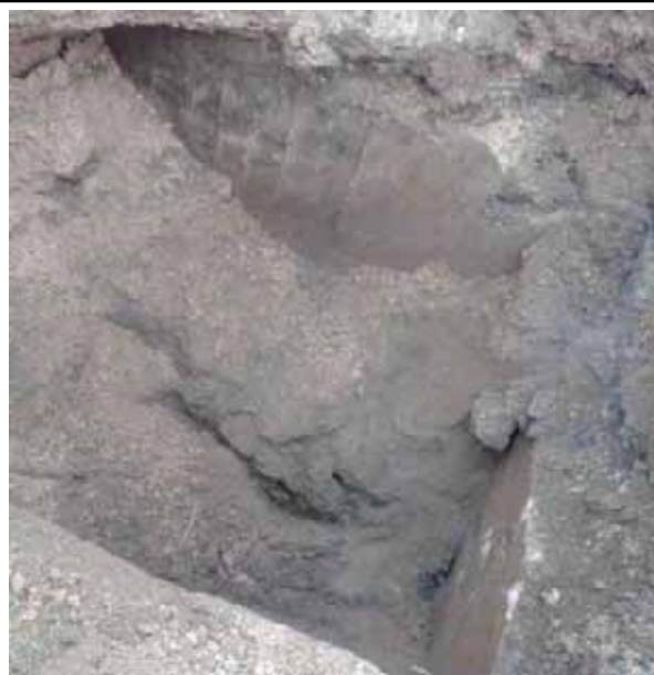
Photograph Twenty - EX301 - Concrete cradle of abandoned tanks visible.
