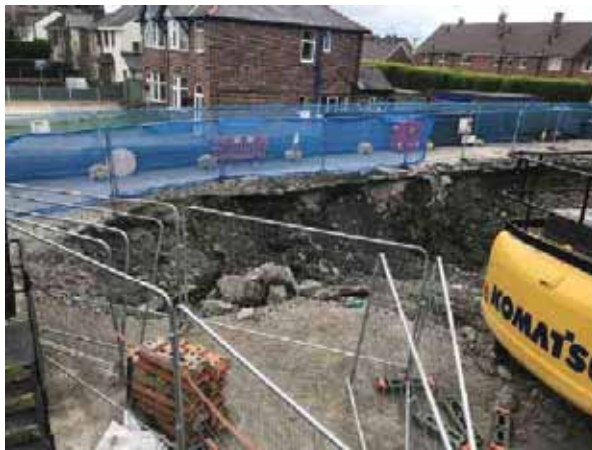
Photograph Five - Excavation remaining in place following removal of the underground tank farm
