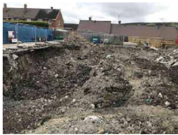
Photograph Six - EX001 (former tank farm) looking south
