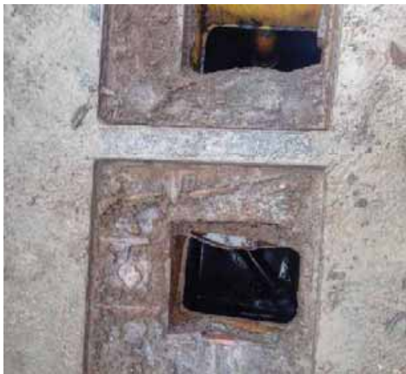
Photograph Twenty-Two - Forecourt interceptor empty and ready for removal.
