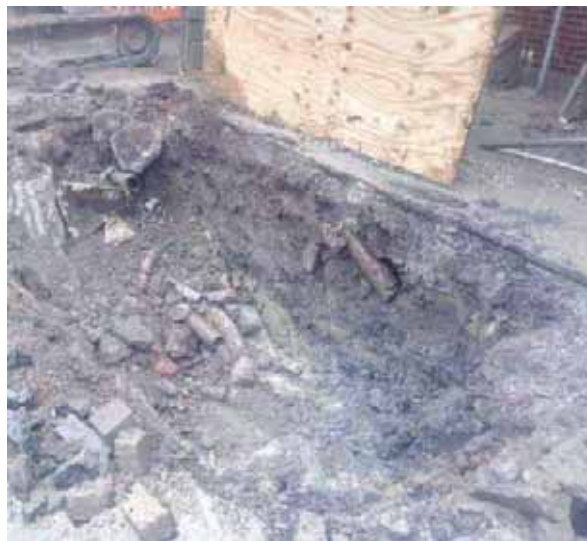
Photograph Twenty-Three - Interceptor being removed. Western wall visible
