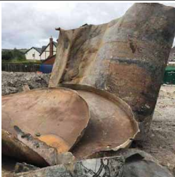
Photograph Seven - Underground tanks removed from EX001
