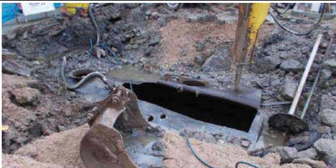
Photograph Thirty-Three- Fifth abandoned tank being cleaned and emptied before removal
