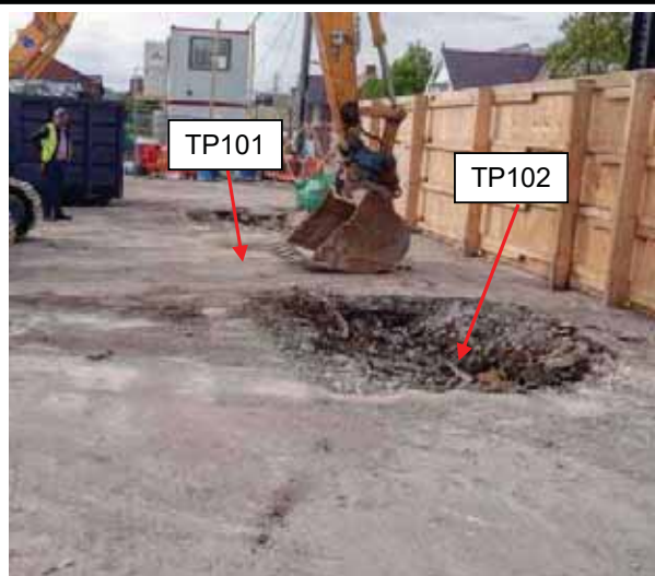
Photograph One - Two trial pits located at the front of the site in the former pump island locations.
