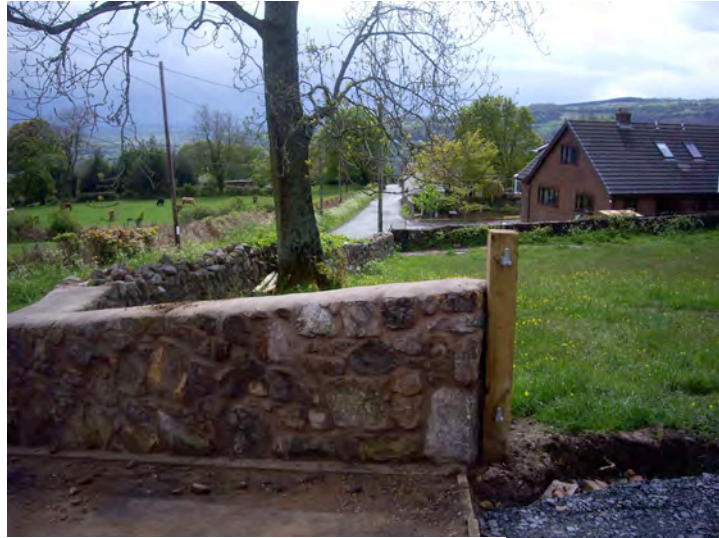
New boundary wall to site entrance
