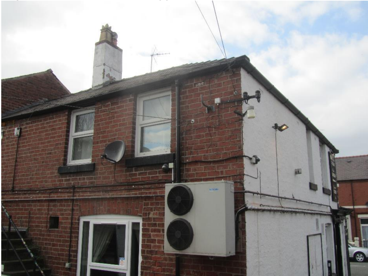
Image 3.16 Southeast corner of B1, showing general construction
