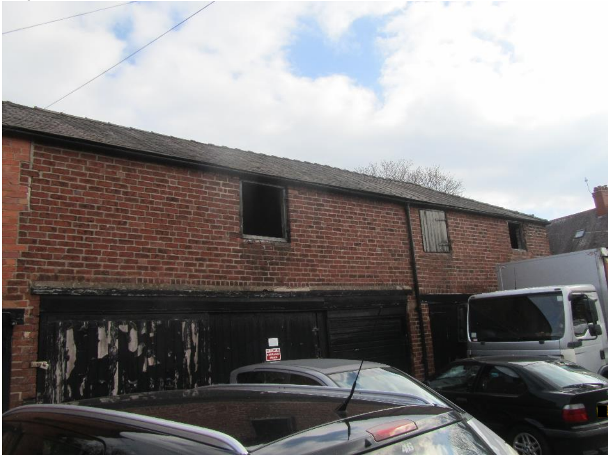
Image 3.26 Northern elevation of B3
