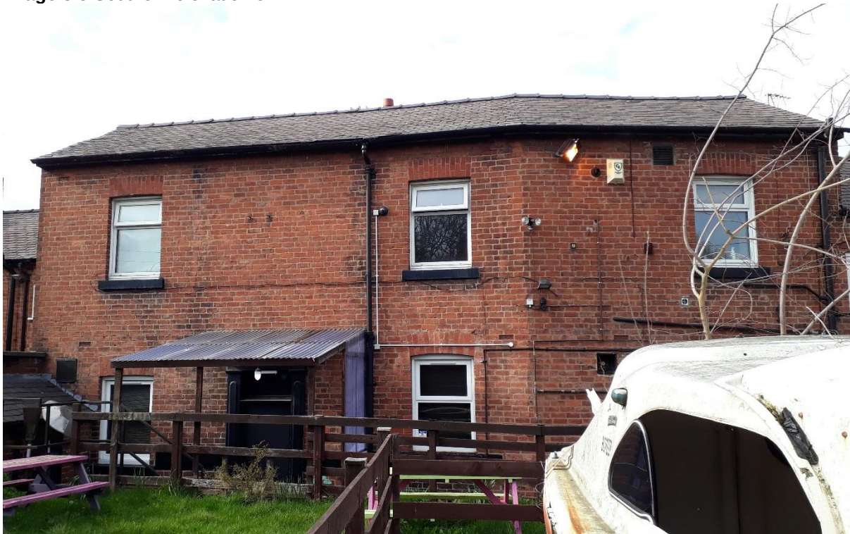
Image 3.5 Southern elevation of B1
