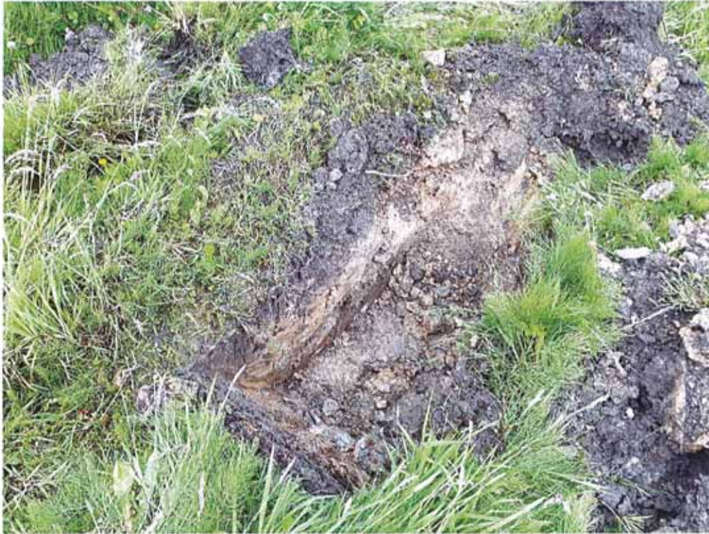
TP E – Pit walls
