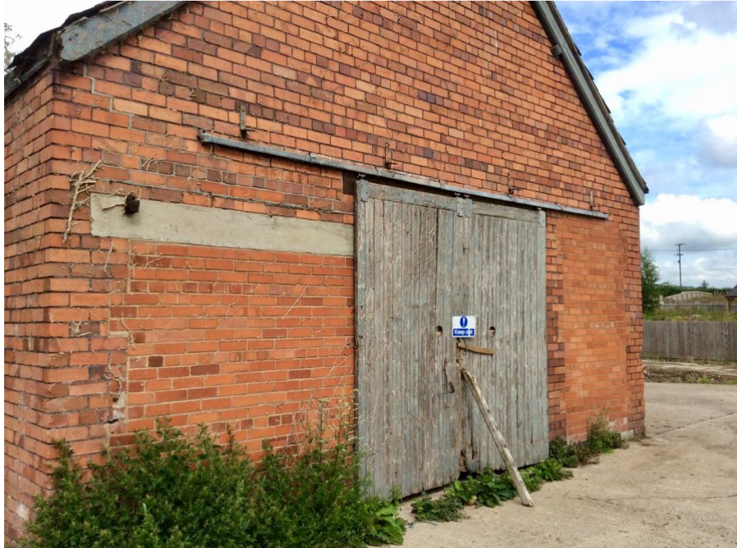
Photo 4 – Existing east elevation
