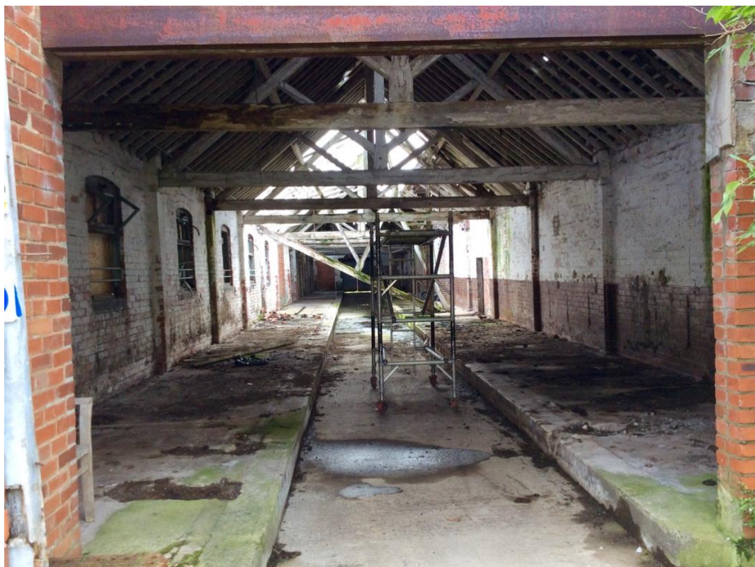
Photo 3 – Inside the main outbuilding
