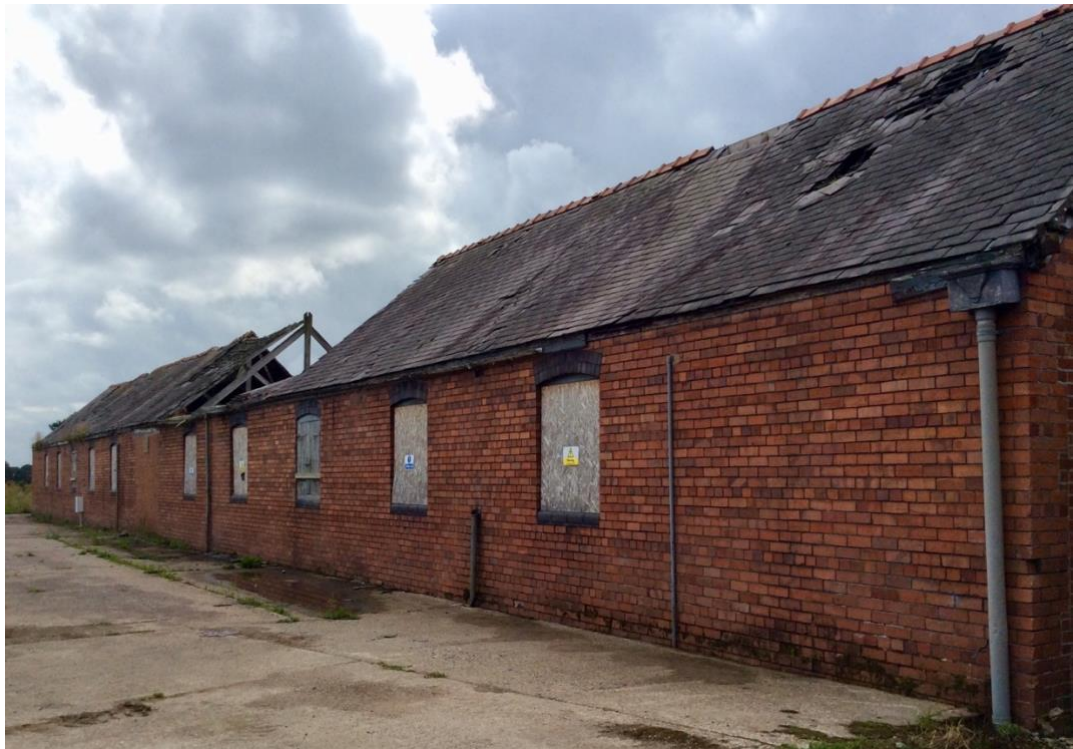
Photo 2 – Main outbuilding existing front elevation
