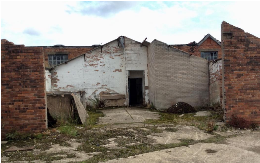
Photo 5 – Part of outbuilding to be demolished
