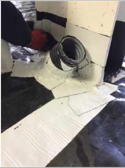
Pipe penetration detail being sealed with detailing tape.
