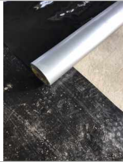
Correct amount of lap being applied.
