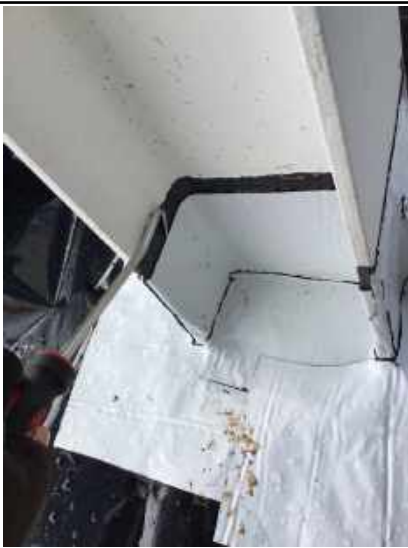
Pick probe testing being carried out
