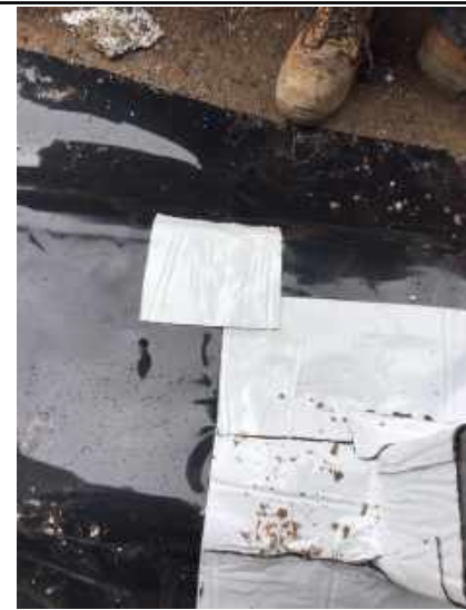
Patch work carried out to the fault
