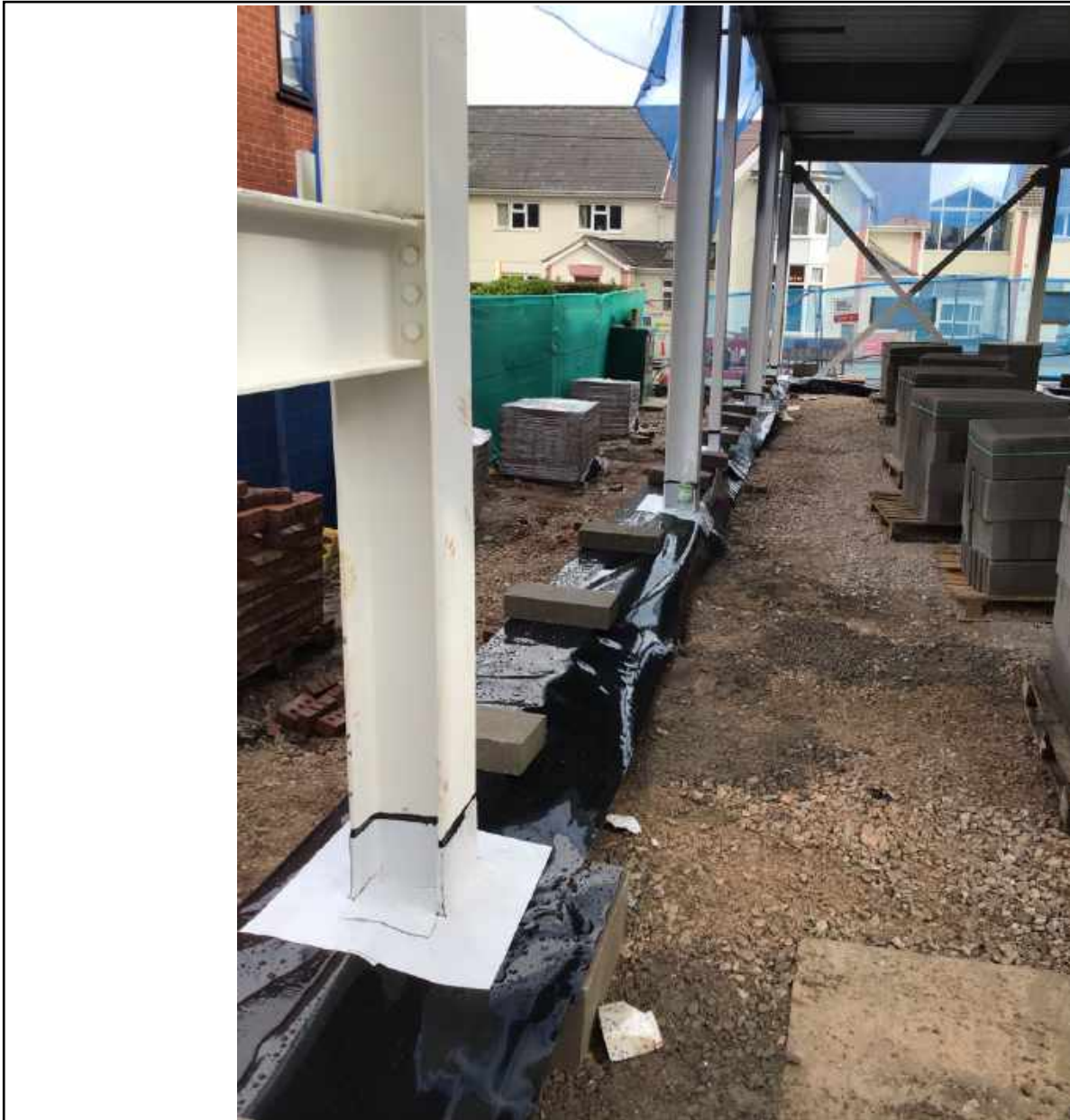
Overview photo looking down the perimeter detail.
