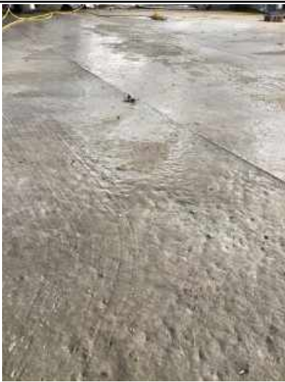
Close up showing that the surface is free from any obstructions.
