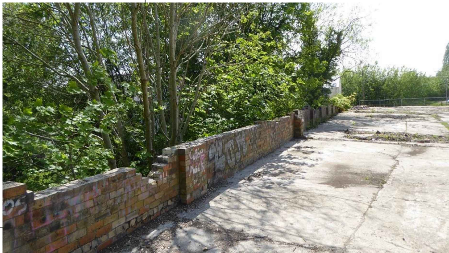
Photo looking towards east of site
