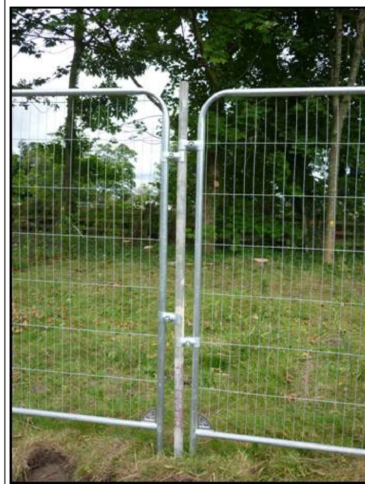
Tree Protective Fencing Specification
