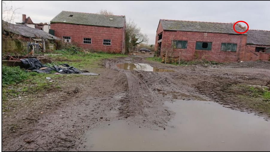
Emergence point at Building 6 during dusk - from crevice in brickwork at wall plate
