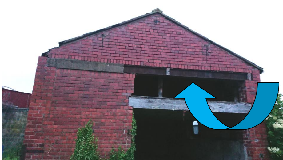
Re-entry point at Building 6 during dawn survey - into mezzanine upper floor and to ridge
