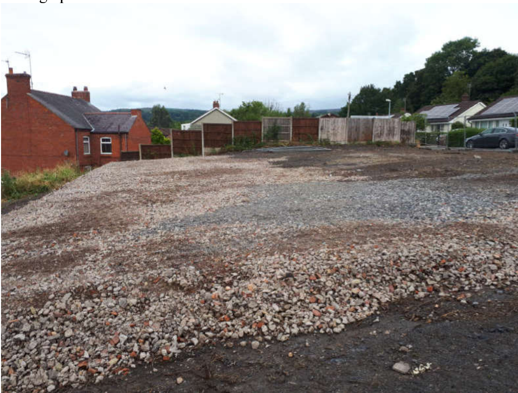
Photograph 2 level platform for drilling and grouting works
