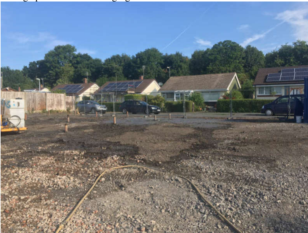
Photograph 2 Grout casings in Plot 1
