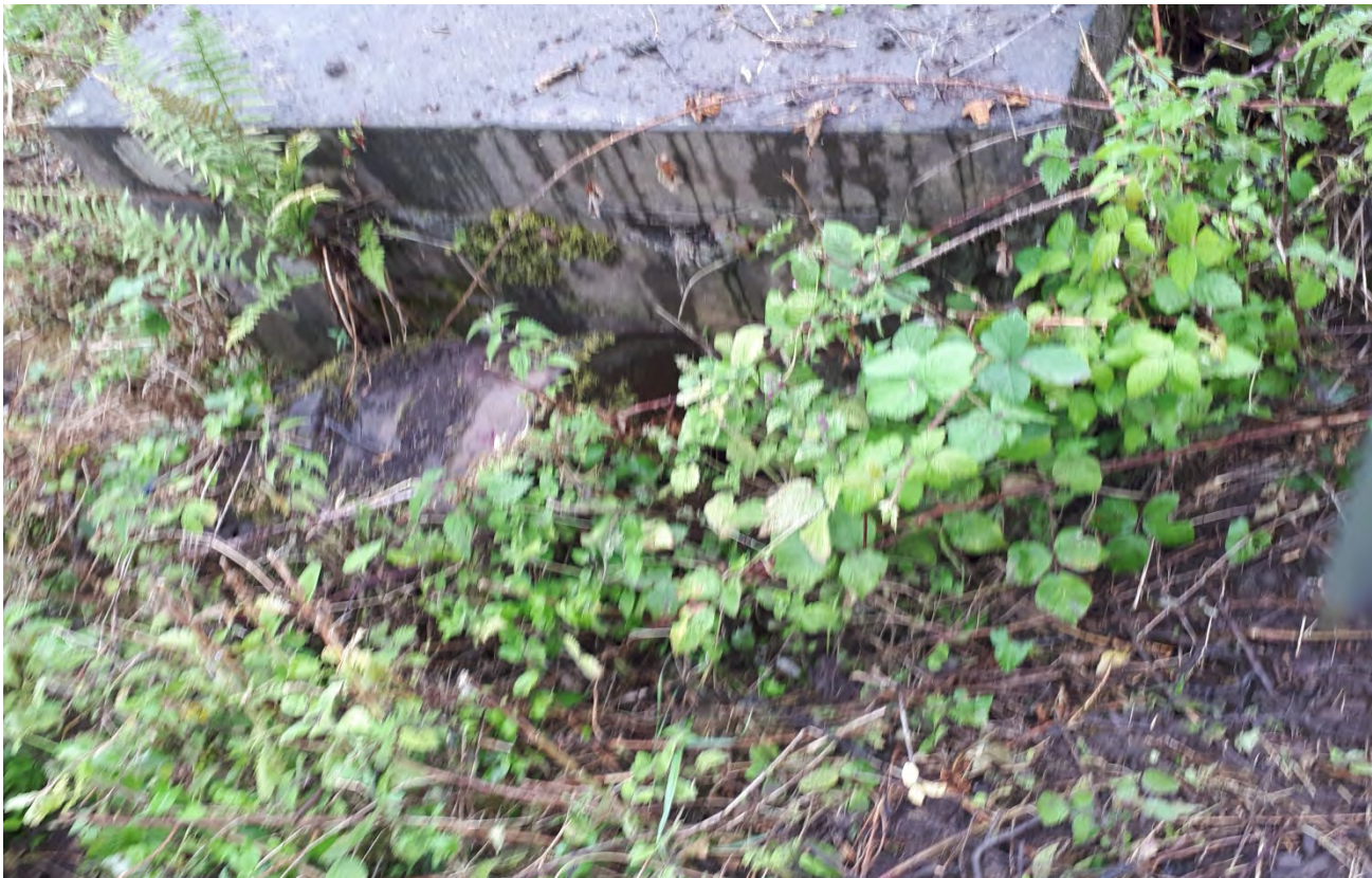
Unknown drum adjacent to north of concrete service cover
