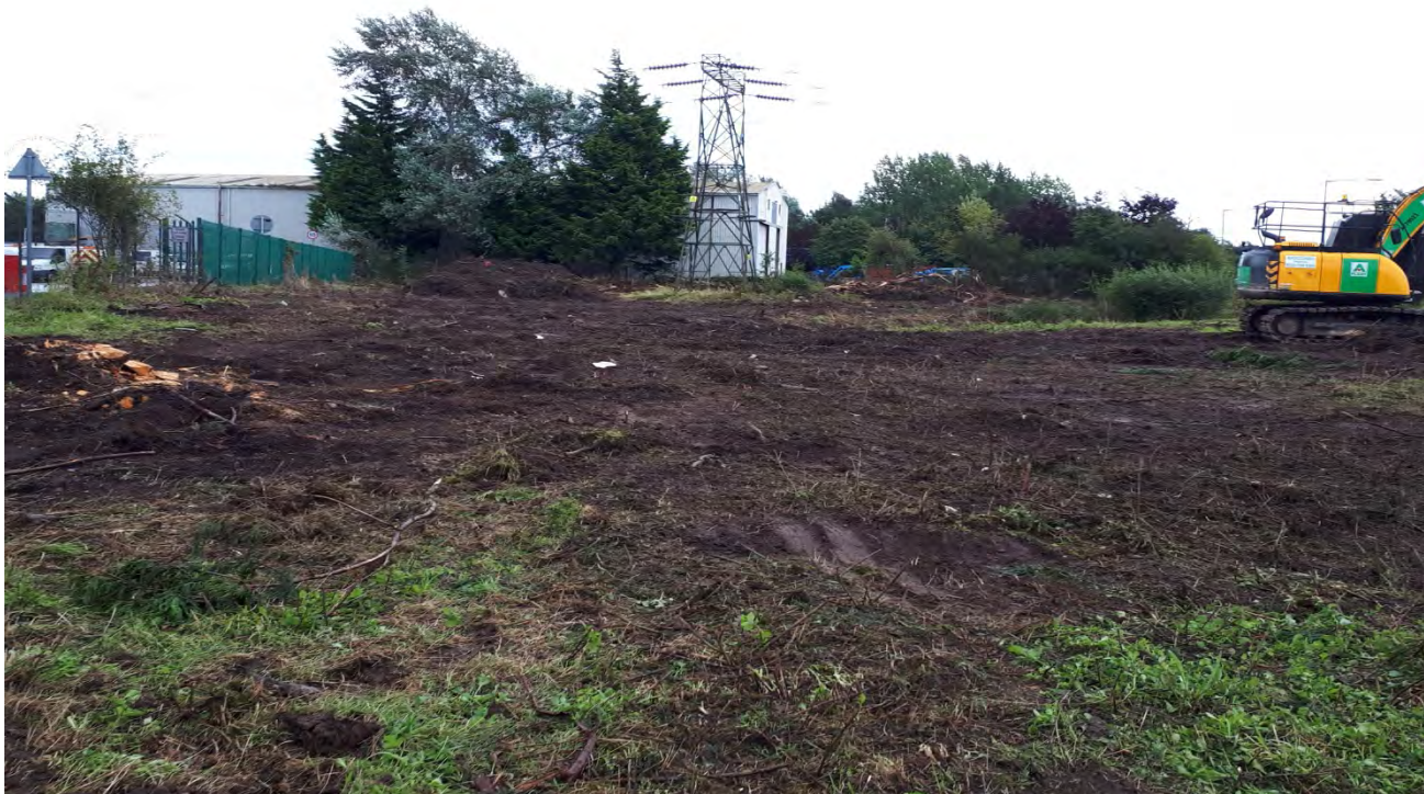
View East along northern boundary towards OHL tower
