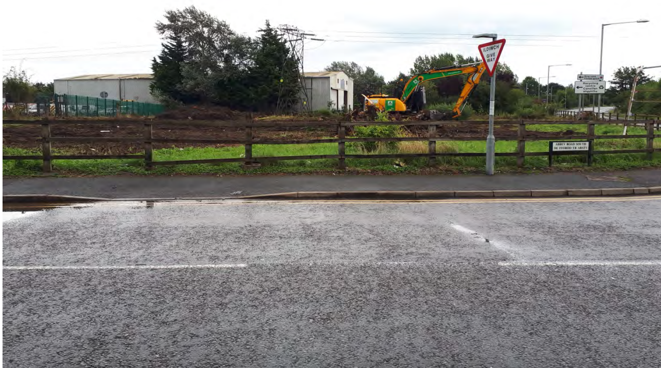
View East from Abbey Road South towards site. Excavator on site – not operating at time of walkover.
