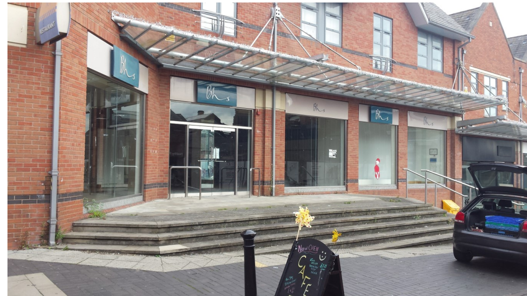
EXISTING PHOTOGRAPH OF SIDE ENTRANCE
