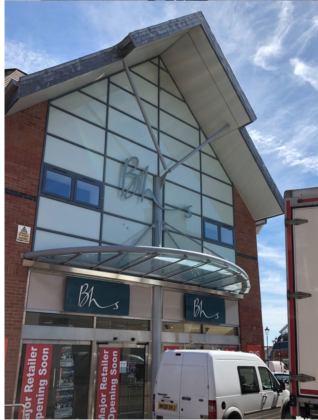
5 EXISTING STORE PHOTOGRAPHY | FRONT VIEW SCALE 1:100 @ A1
