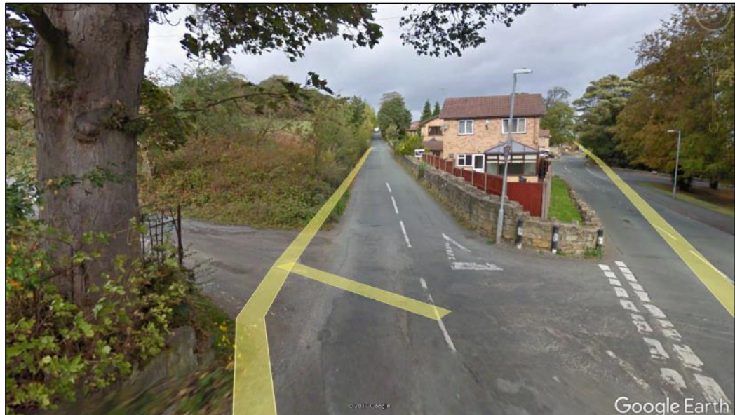
Figure 2.1 – View along Top Rd from the Junction of Summerhill Rd/Top Rd/Bottom Rd
