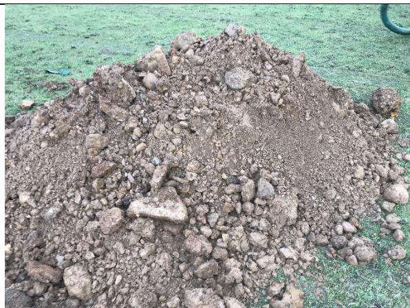
Soakaway Pit 05: Excavation spoil.
