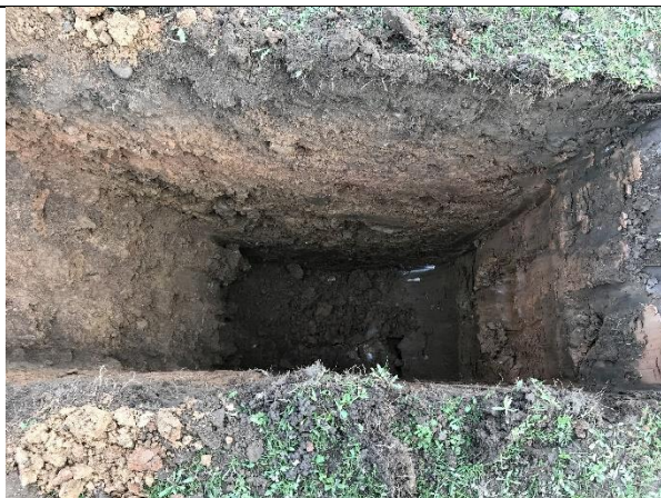
Soakaway Pit 04: Internal view of excavation.
