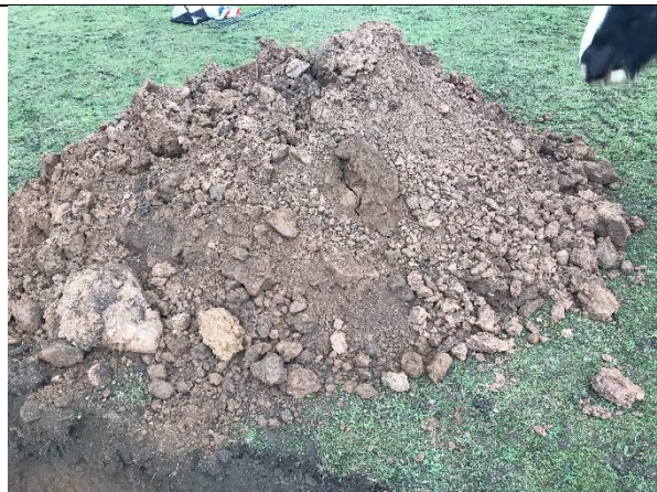
Soakaway Pit 01: Excavation spoil.
