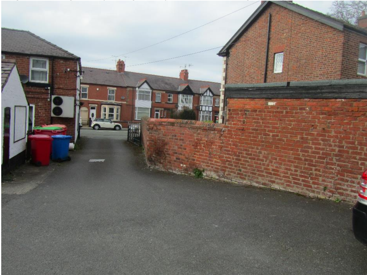
Image 3.10 Existing driveway leading into carpark area, also showing boundary wall
