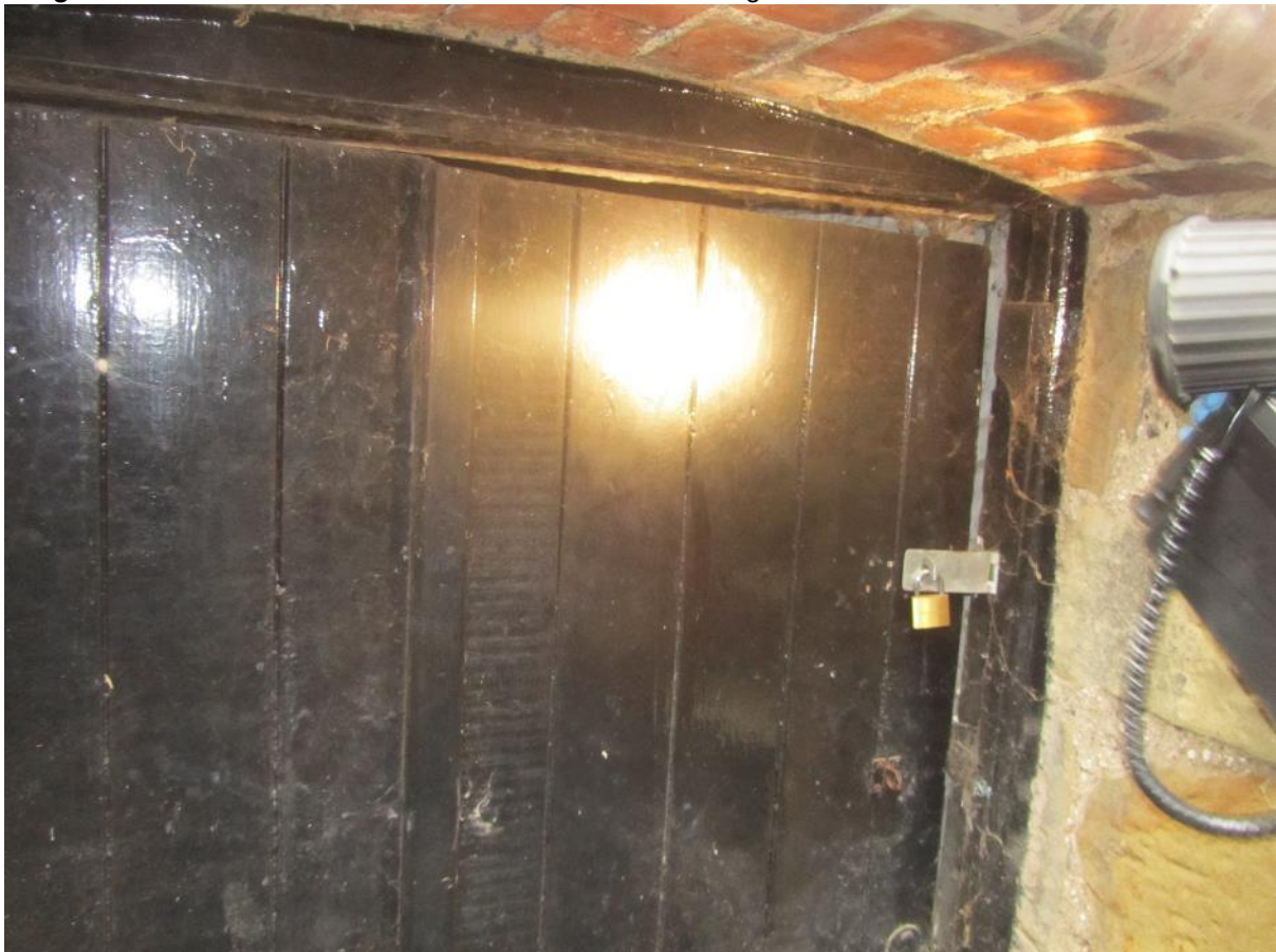
Image 3.21 Basement/ cellar below B1 – inaccessible during the PRA
