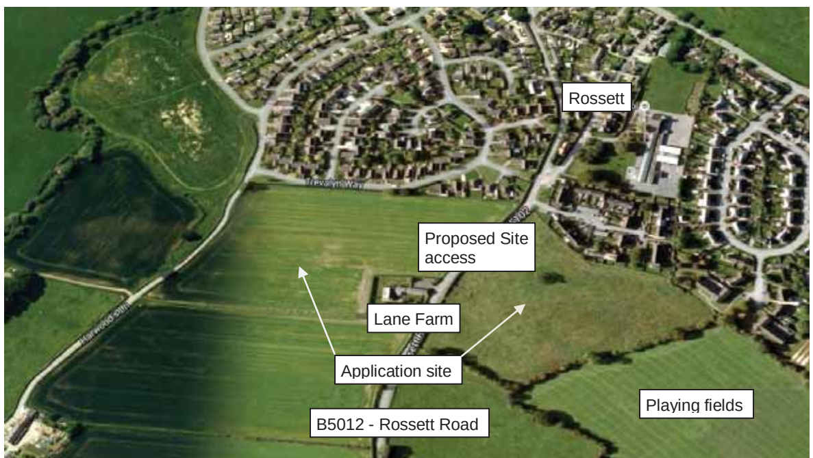
Oblique, elevated view towards application site from north-west
