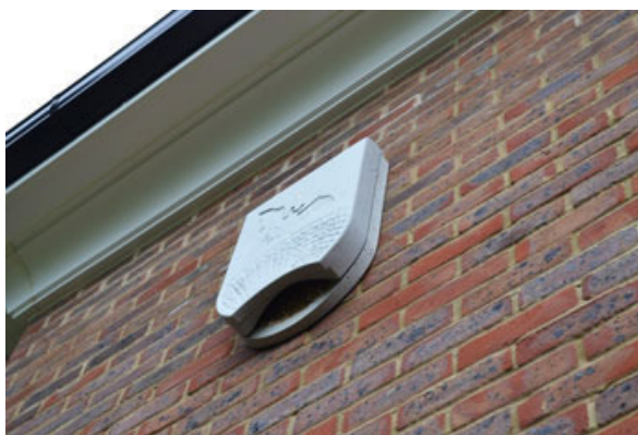
Figure 13: Schwegler (1FQ) bat box fitted to wall.
