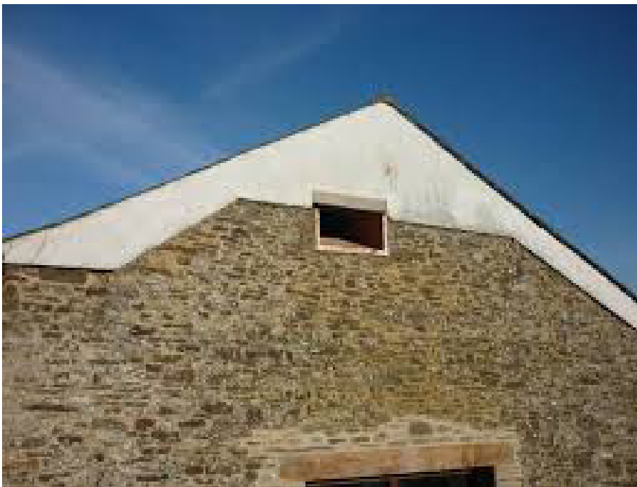
Figure 15: Example of LHS fly in access in gable-end wall.
