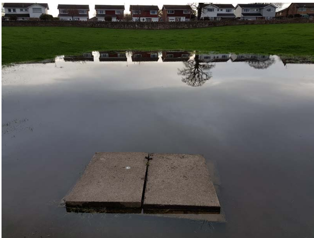
Photo 25 – View of manhole in pond in area 4
