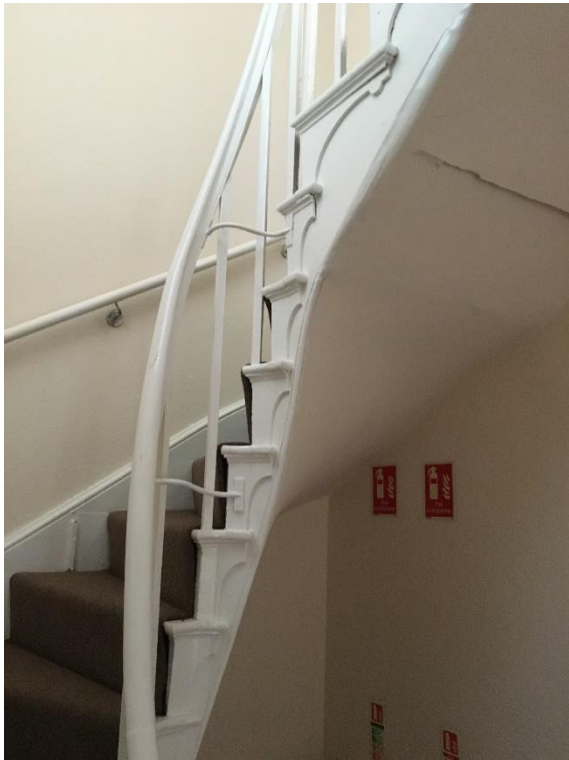
Fig 4-First to Second Floor Stair String
