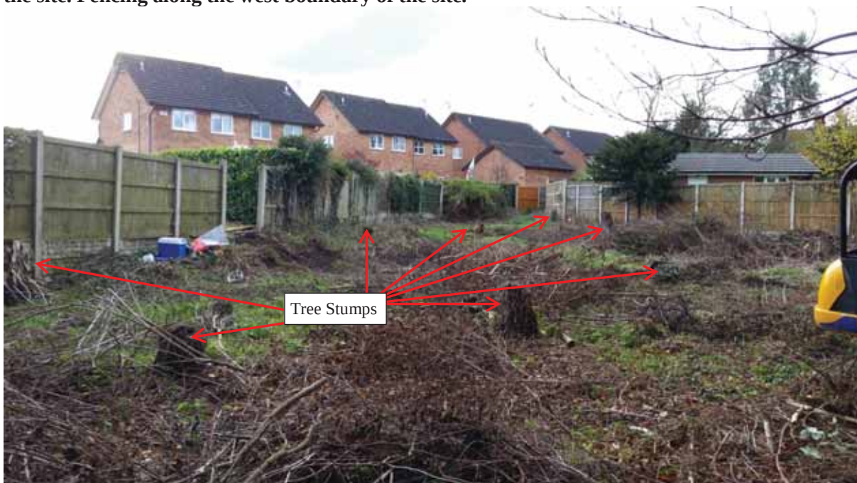
Photograph 4: Taken facing southwest from northeast corner of the site. Shows the shrub covering the site. Fencing along the west and south boundary of the site. Access through the southern boundary fencing which can be removed.
