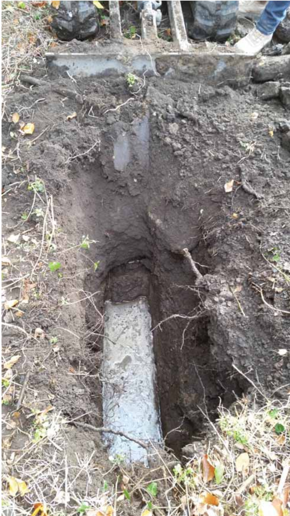
Photograph 23: Shows TP03 to a depth of 2m.
