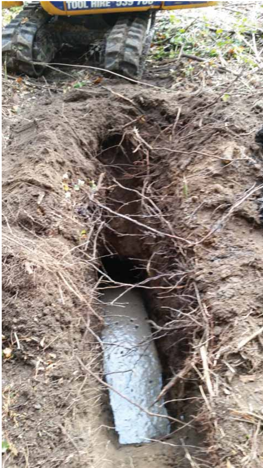
Photograph 25: Shows TP04 to a depth of 2m.
