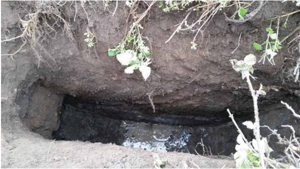
Photograph 16: Shows TP01 and sides of trial pit.
