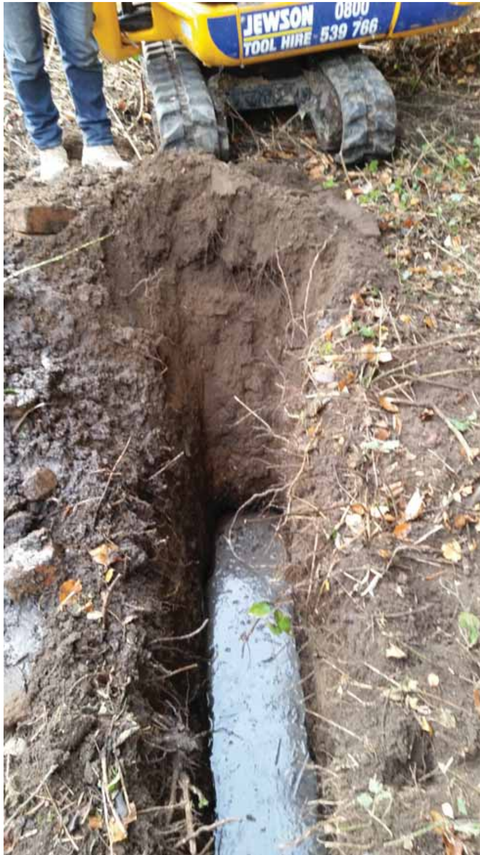
Photograph 30: Shows TP05 to a depth of 2 m.
