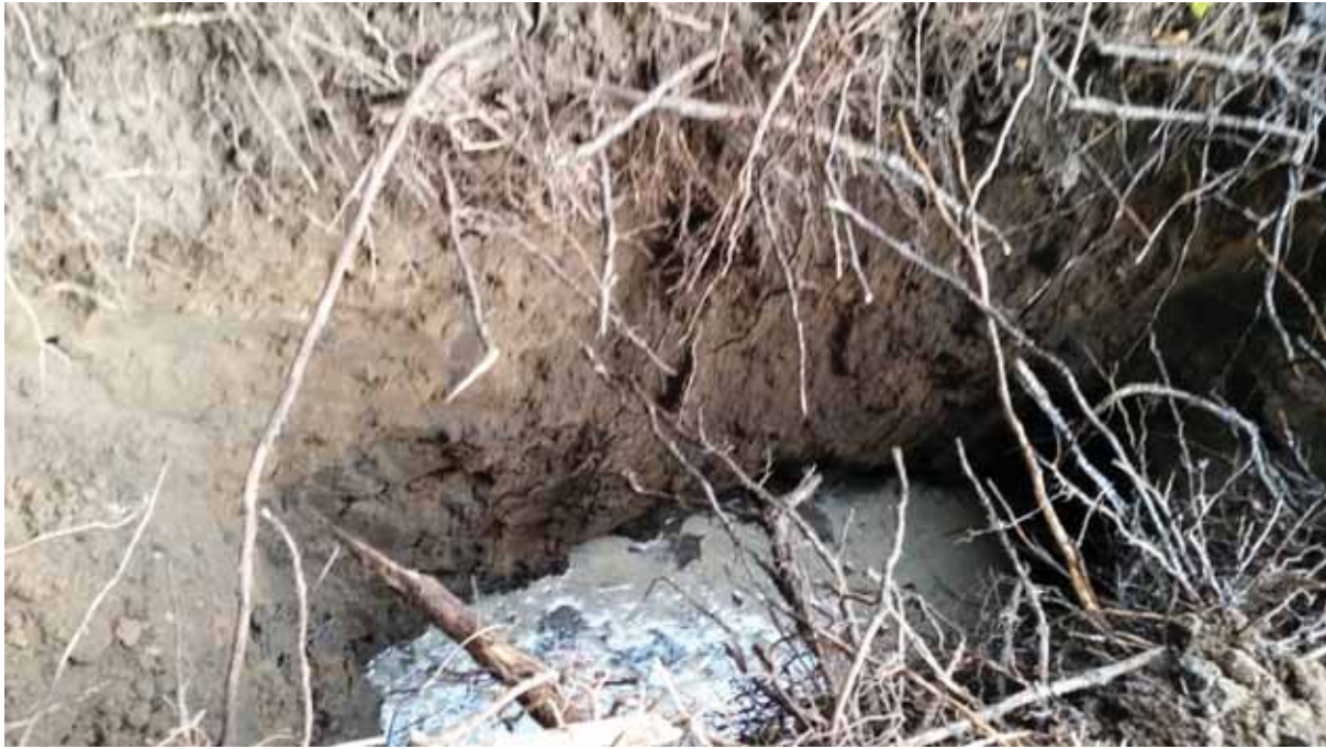
Photograph 28: Shows TP04 to a depth of 2m and the sides of the trial pit.
