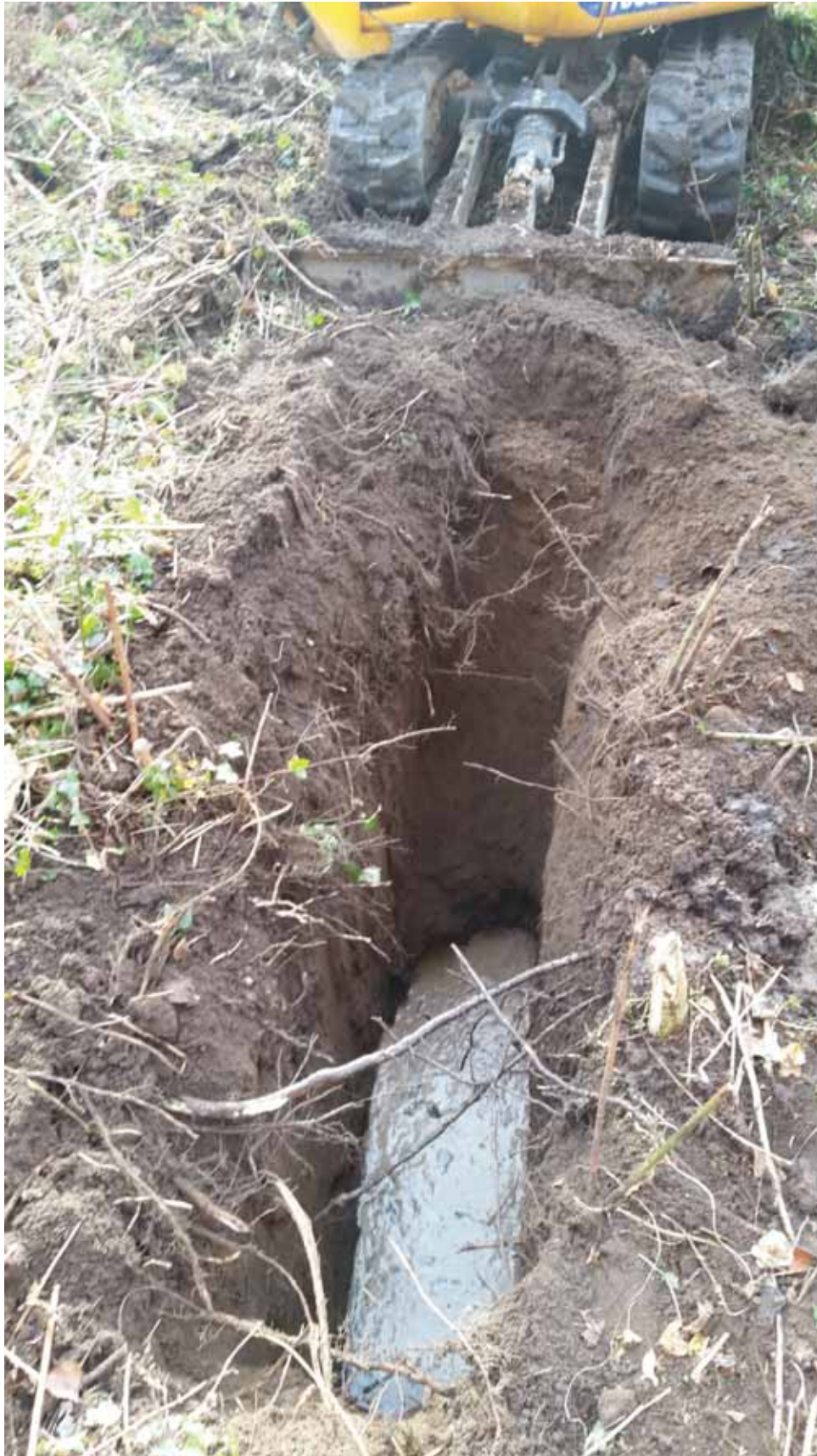
Photograph 20: Shows TP02 to depth of 1.8m.
