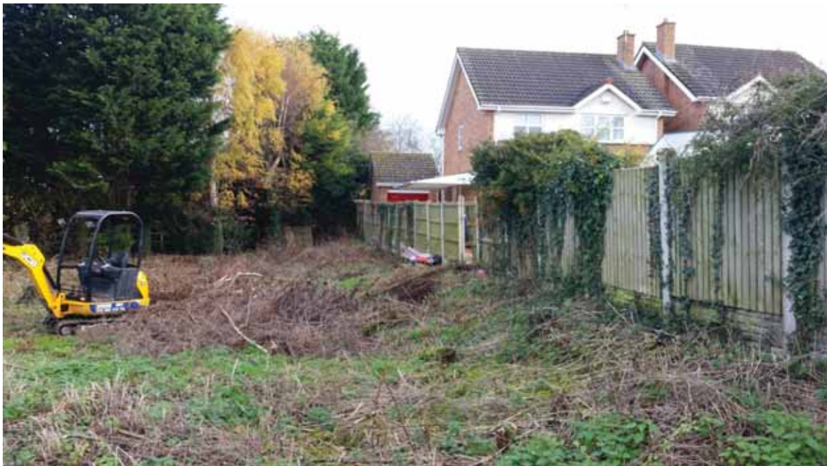
Photograph 2: Taken facing northeast from southwest corner of the site. Shows the shrub covering the site. Fencing along the southern boundary of the site which can be removed for access.
