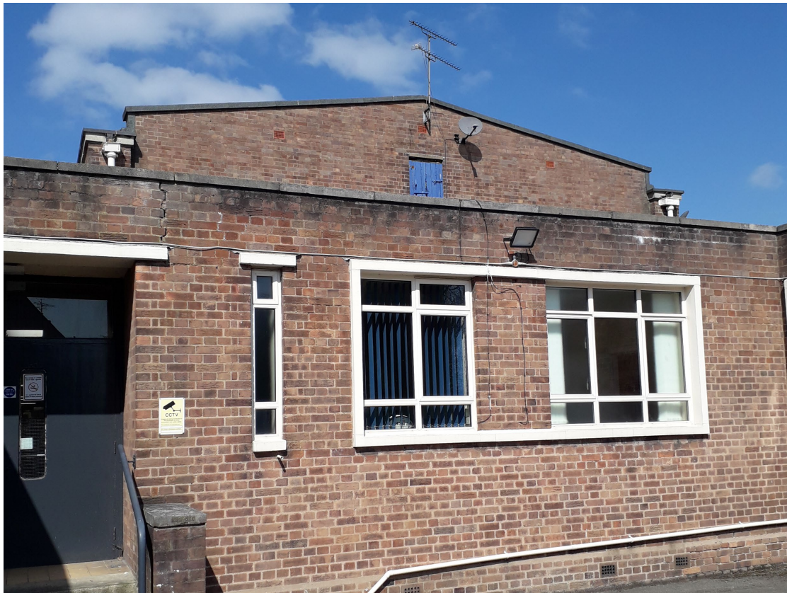
Image EDP 3.1: Building 2 with external access to loft void on south-eastern aspect
