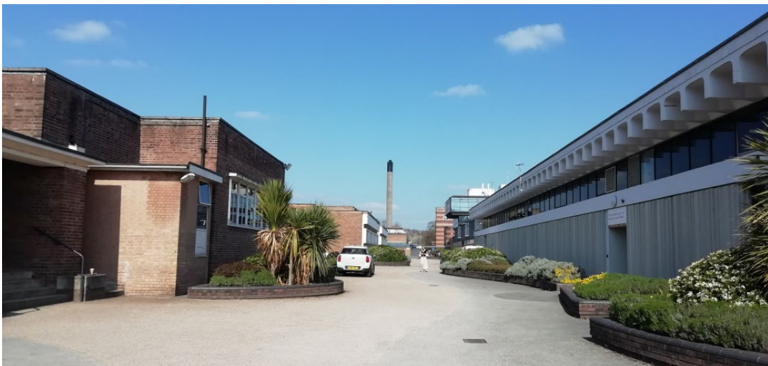
Image EDP A2.2: Buildings 8 and 9 (left) with ornamental shrubs and hardstanding road
