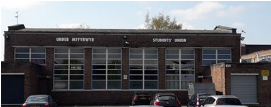
Image EDP 3.2: Building 2 with car parking as viewed on south-western aspect
