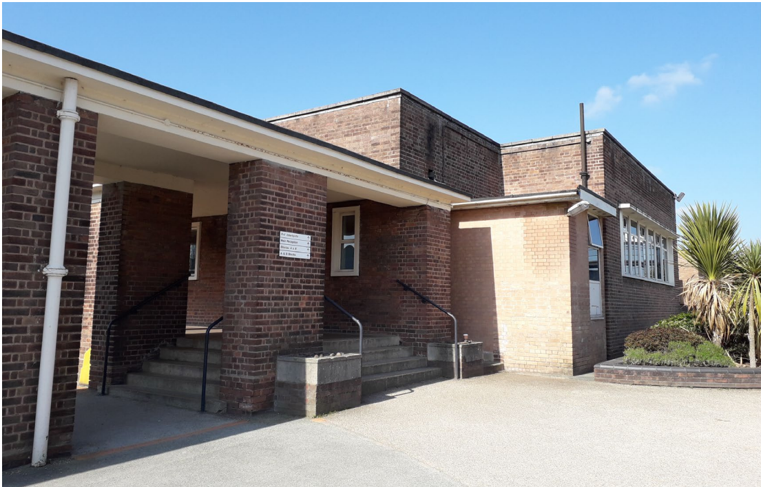
Image EDP 3.3: Building 9 with 'walkway' to Building 2
