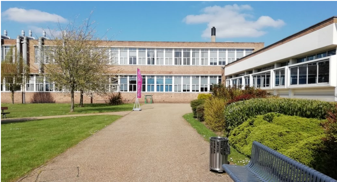
Image EDP A2.1: Building 8 (right) with semi-improved grassland and scattered trees in the student garden (left)
