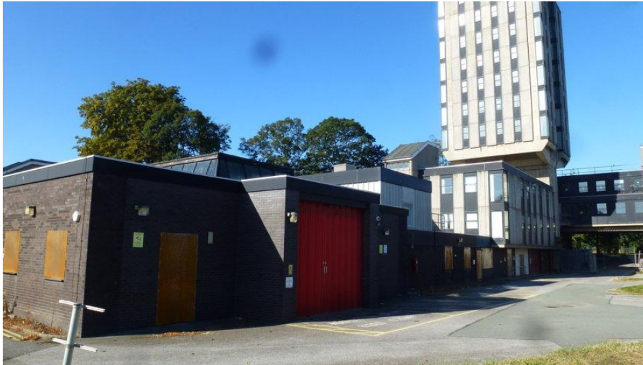
Photograph 1: General view of eastern frontage to site. Note: The police station buildings including the multi storey tower to rear, garages and utility buildings and hard standing to fore.
