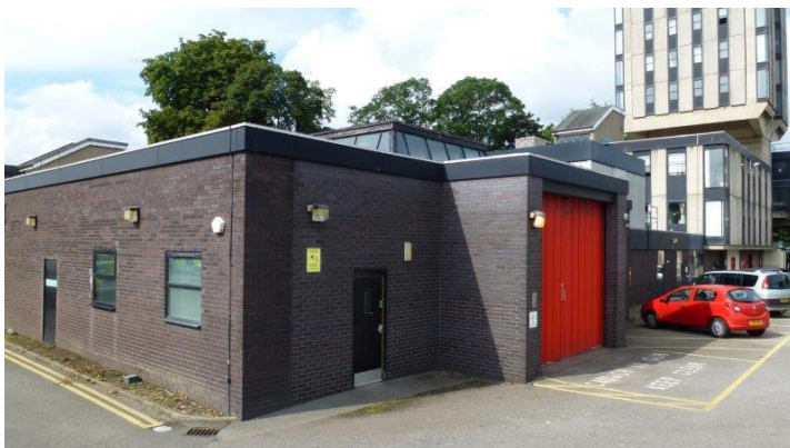
Photograph 7: View of low level vehicle garage annexe building.
