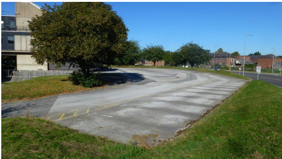
Photograph 2: View from south east corner of site showing grass covered screening embankment, extensive hard standing parking provision, and busy highway to right of image.
