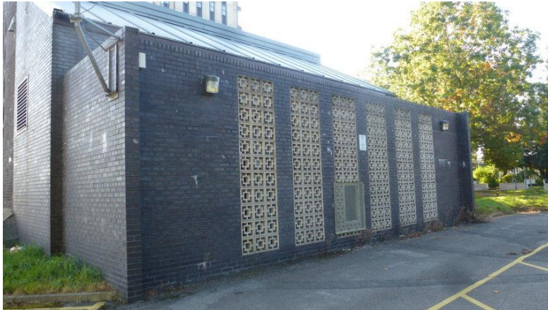
Photograph 8: View of ornamental facade screening to service building.
