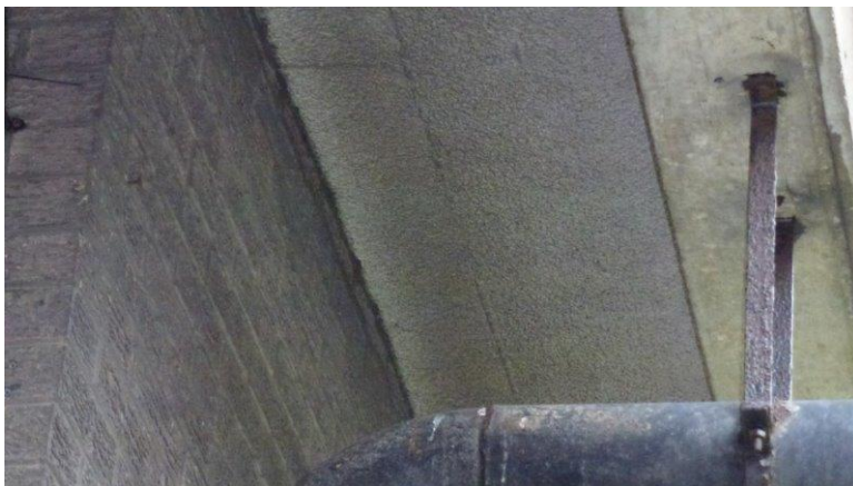
Photograph 9: Close up view of typical concrete roof overhang. Note well sealed against wall.
