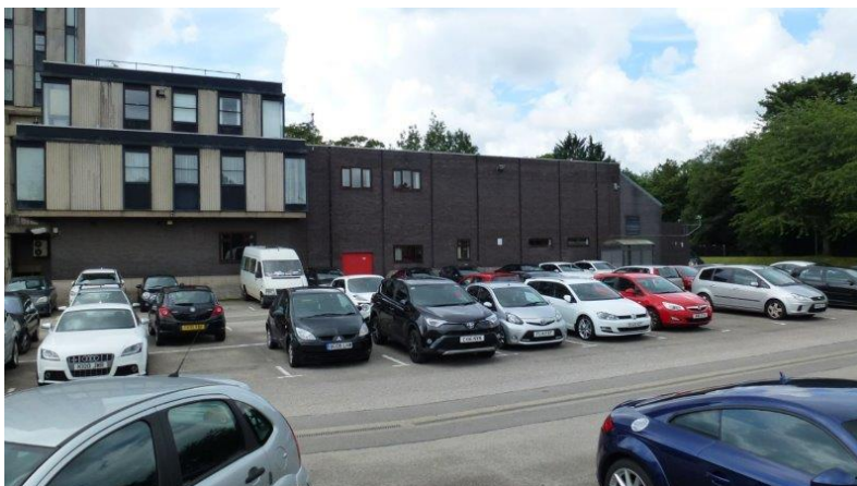
Photograph 4: View of east frontage low level buildings.
