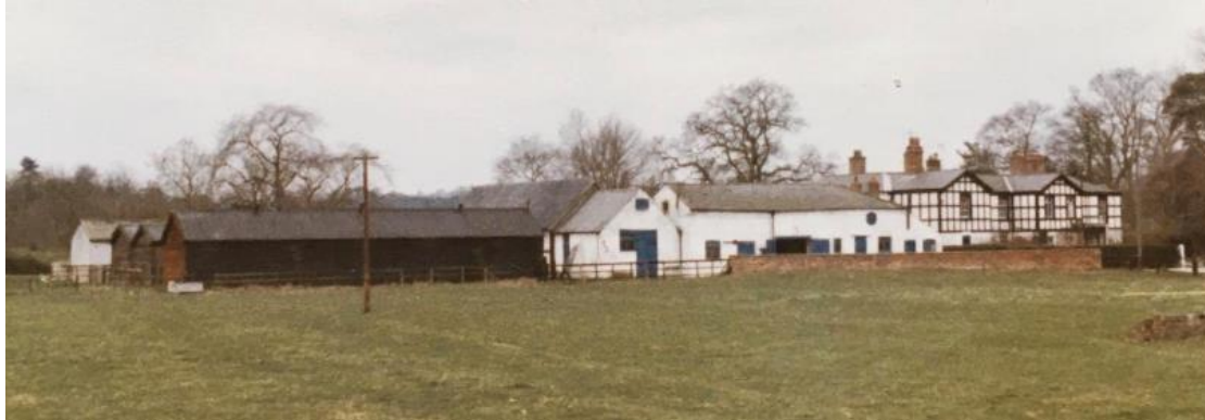
Photograph showing north elevation including farm buildings, circa 1970's
