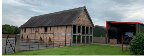
Existing west elevation also showing listed barn
