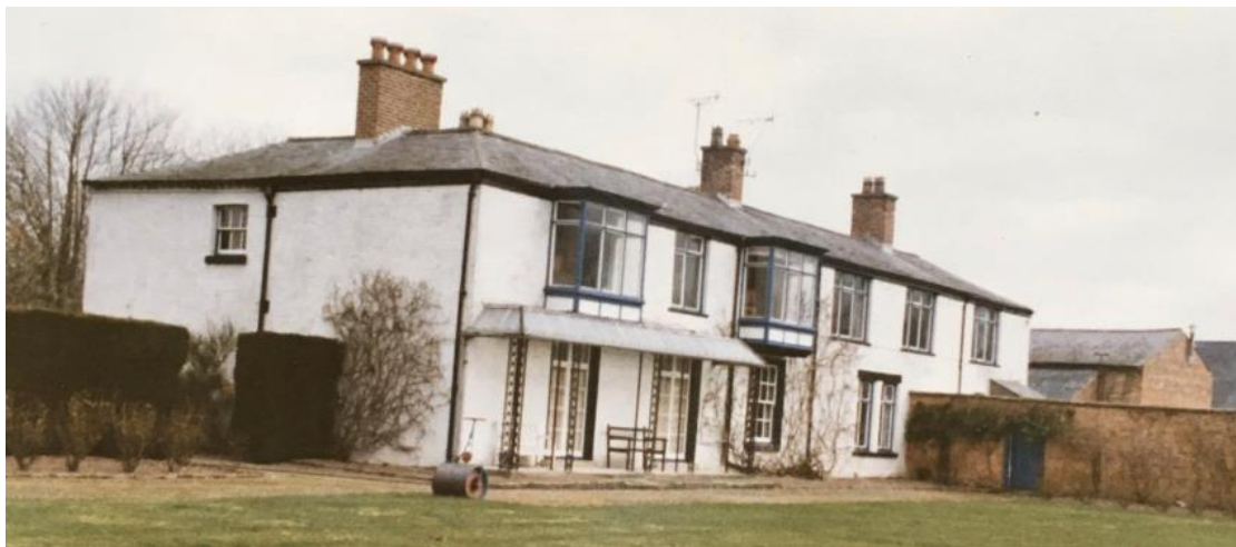
Photograph showing south elevation, circa 1970's
