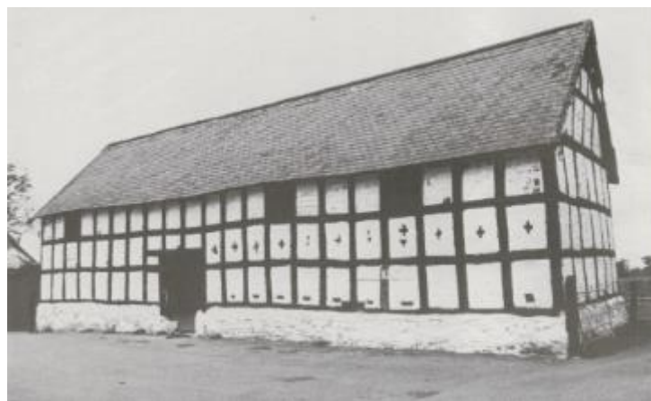
Example of timber framed building in Ruthin Source: The Historical Farm Buildings of Wales Eurwyn Wiliam
