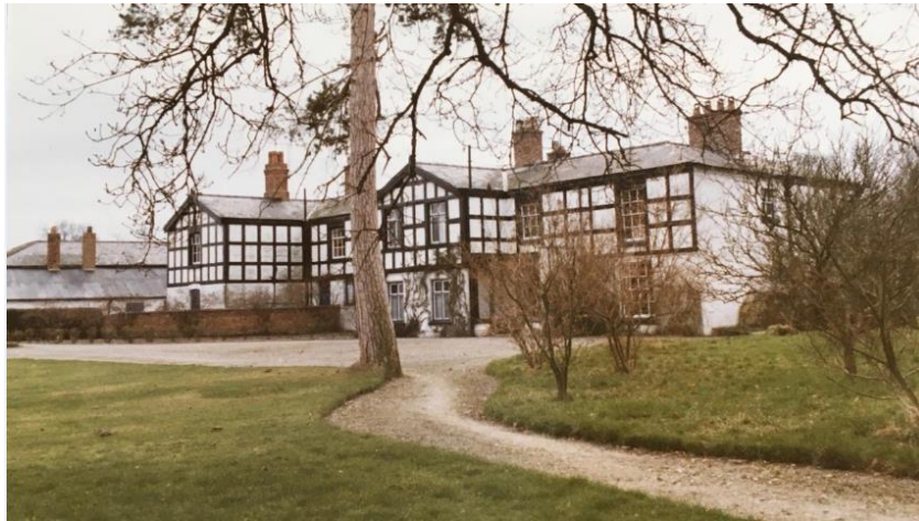
Photograph showing north elevation, circa 1970's
