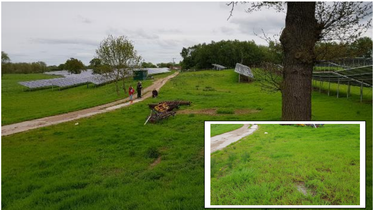
Figure 7: Area of waterlogging near the west Inverter set (#1)
