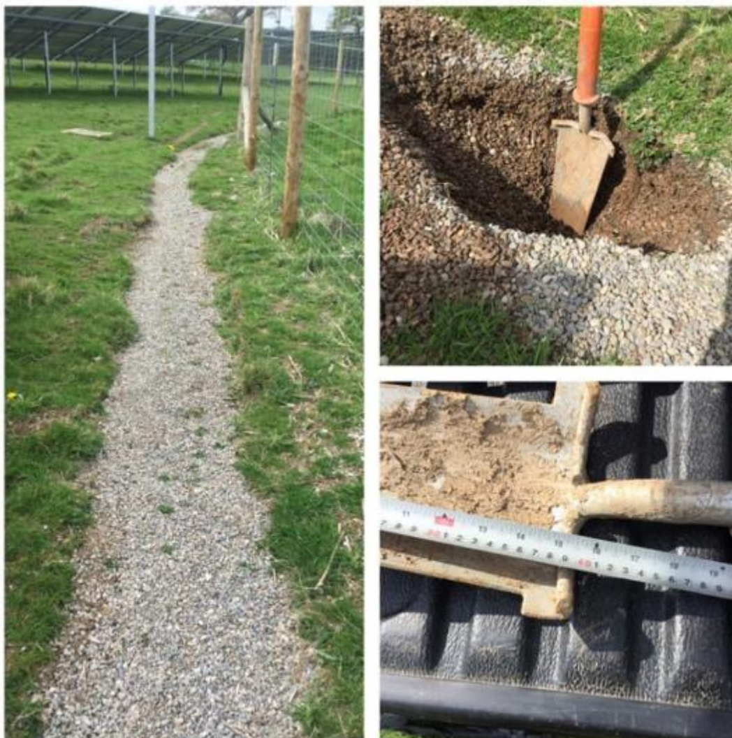
Figure 17: Gravel trench – Section CD
