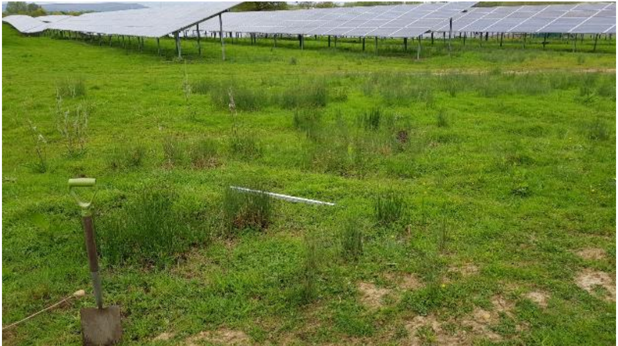
Figure 8: Area of waterlogging in west field near southern boundary
