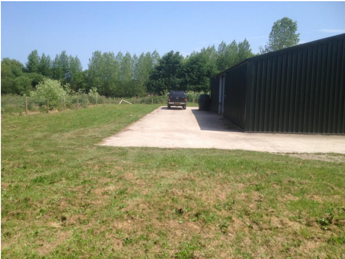
Plate 1: View of the concrete apron that covers much of the proposed development site
