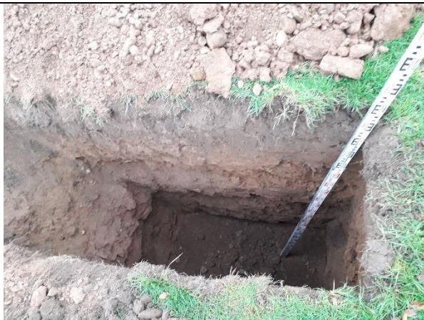
Soakaway Pit 07: Internal view of excavation.
