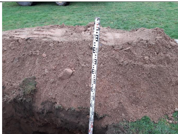
Soakaway Pit 08: Excavation spoil.
