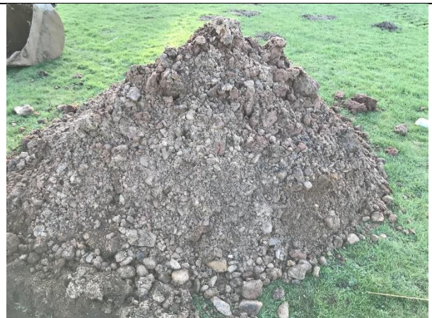
Soakaway Pit 10: Excavation spoil.
