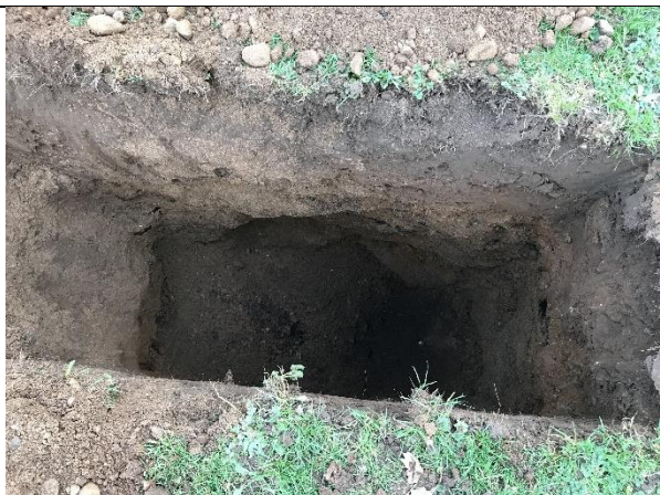
Soakaway Pit 06: Internal view of excavation.
