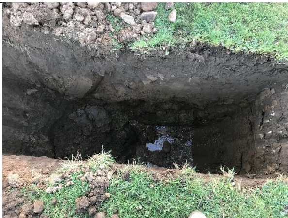
Soakaway Pit 10: Internal view of excavation.
