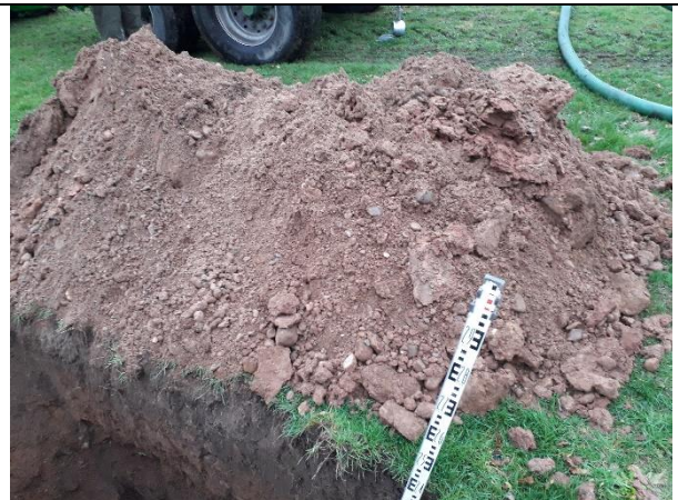
Soakaway Pit 07: Excavation spoil.
