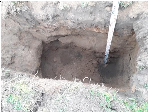
Soakaway Pit 08: Internal view of excavation.
