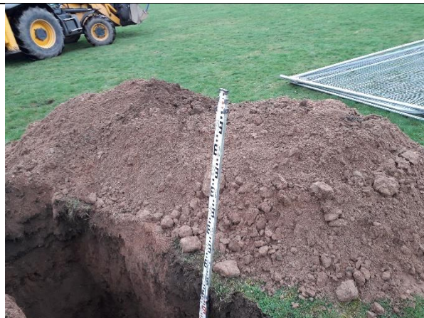
Soakaway Pit 09: Excavation spoil.
