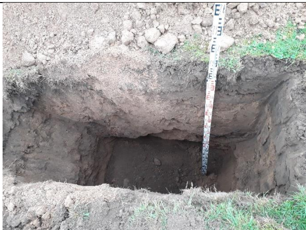
Soakaway Pit 09: Internal view of excavation.
