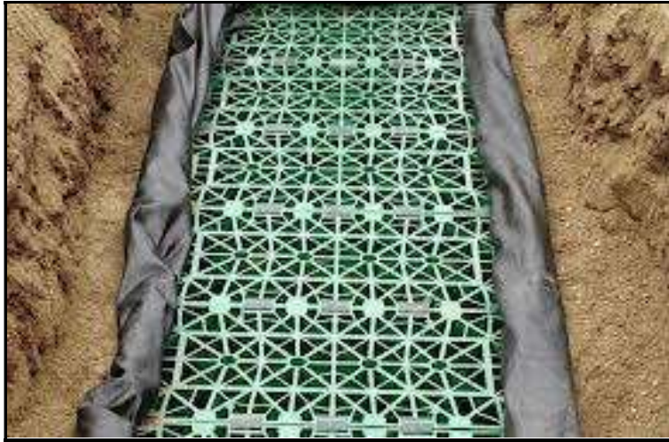
Figure 11: Soakaway trench
