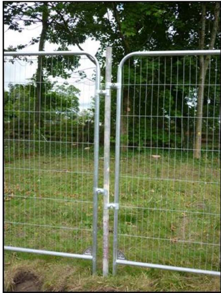
Tree Protective Fencing Specification
