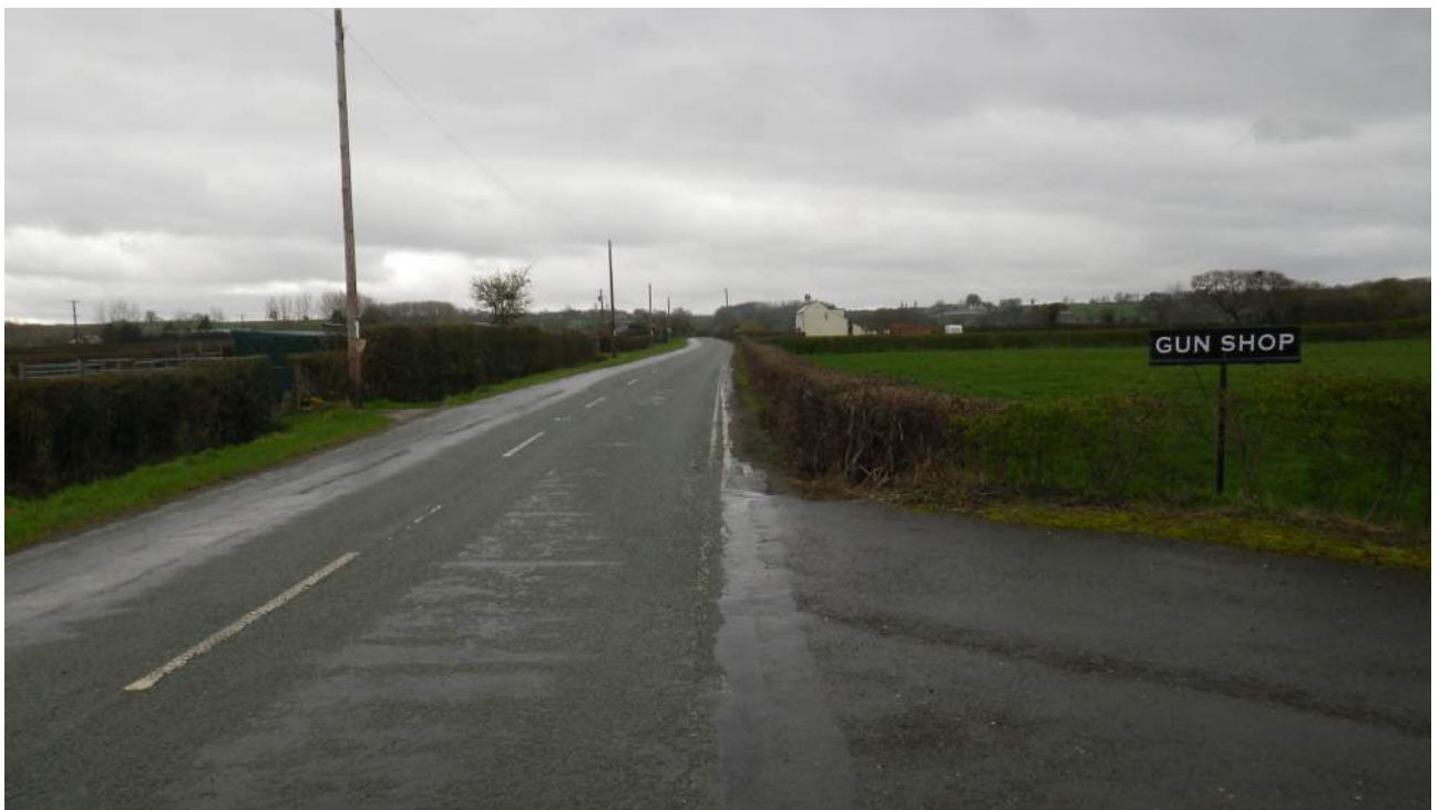
PHOTOGRAPH 2 From road channel looking west
