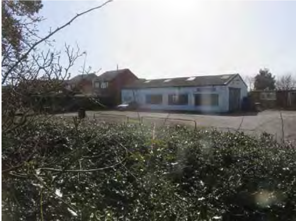
Photo 41 – View of former vehicle repair workshop on across Gresford Road from the southwestern site boundary
