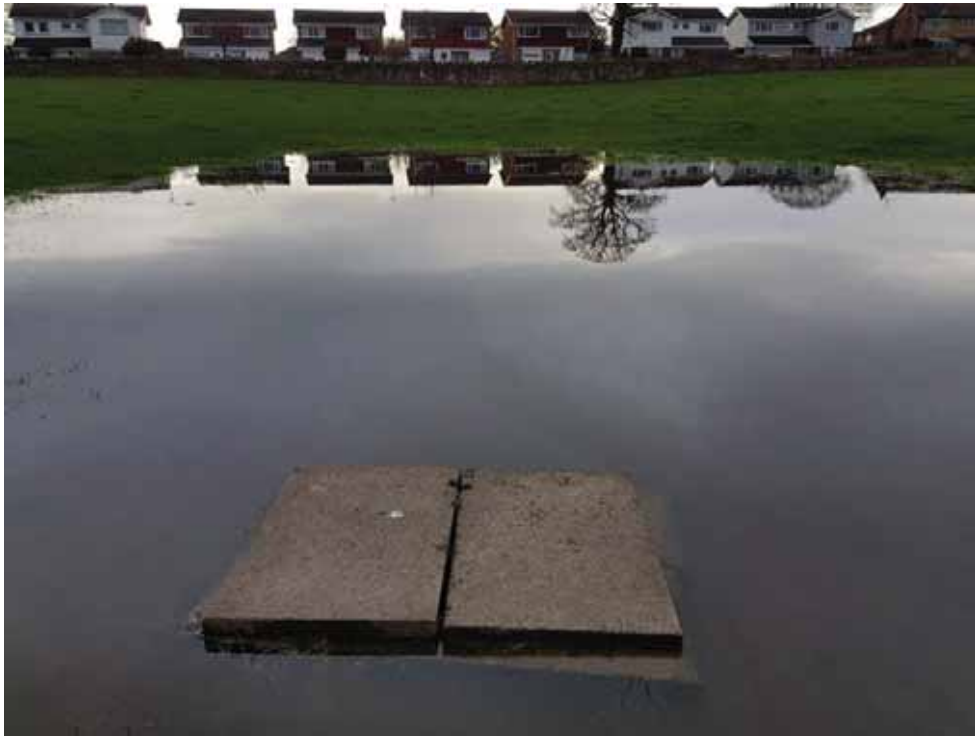
Photo 25 – View of manhole in pond in area 4
