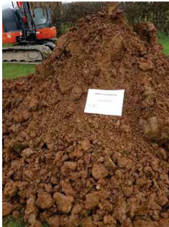
Photo 4 – Arising's Trial Pit 02
