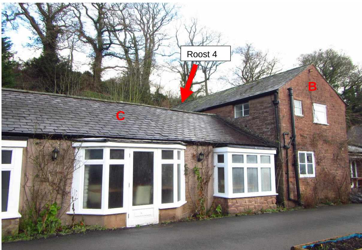
Photo 6. Front (south) elevation of Building B and Building C.
