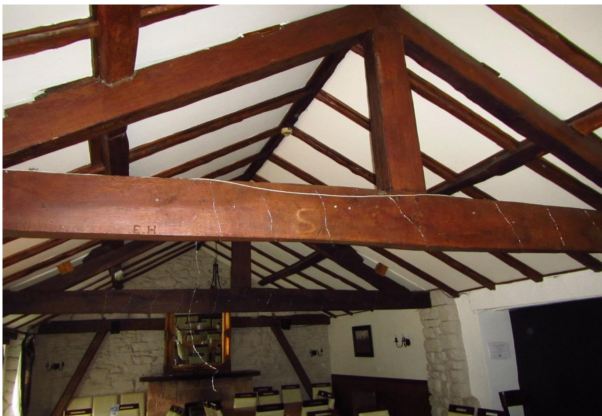
Photo 12. Interior of Building C.
