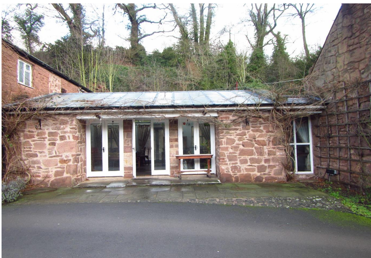
Photo 10. Front (south) elevation of Building D connecting A and B.
