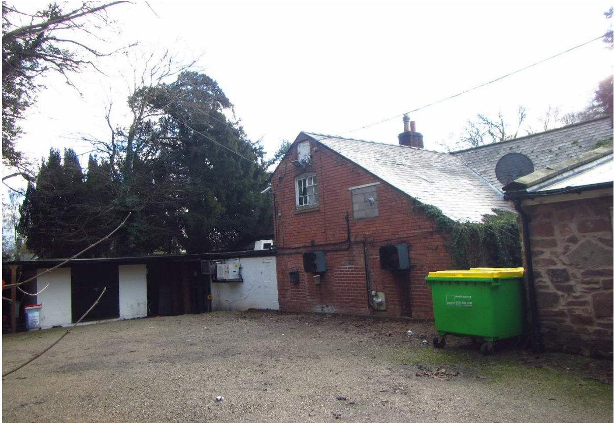
Photo 5. Rear (north) of Building A.
