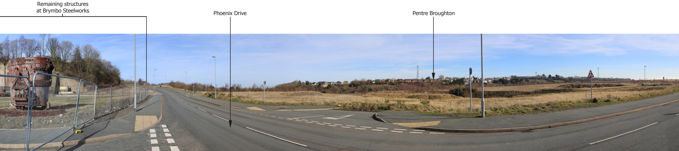
SITE APPRAISAL PHOTOGRAPH C: VIEW NORTH-EAST FROM PHOENIX DRIVE ADJACENT TO BRYMBO STEELWORKS RETAINED STRUCTURES
