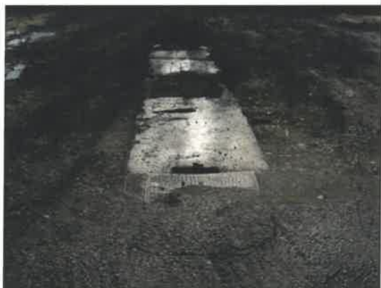
Underground storage tank(s)
