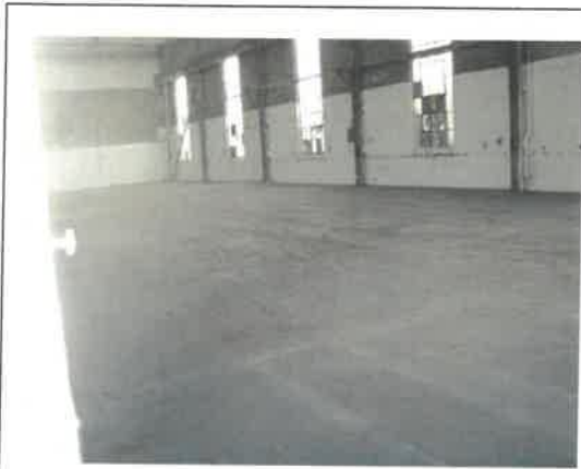
Internal area to Unit 226D
