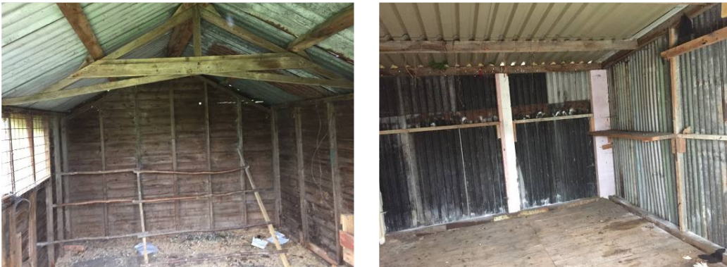
Plate 7: Interior of outbuildings
