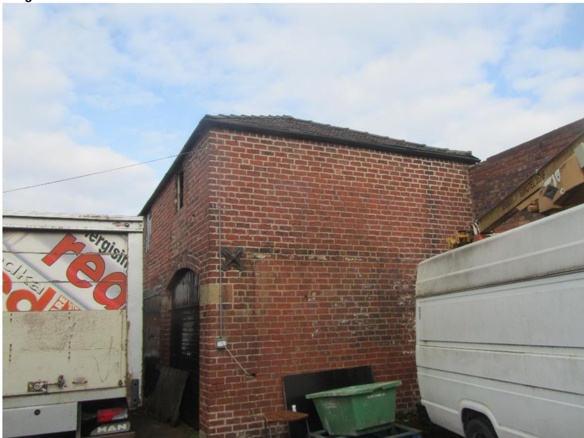
Image 3.25 Western elevation of B3
