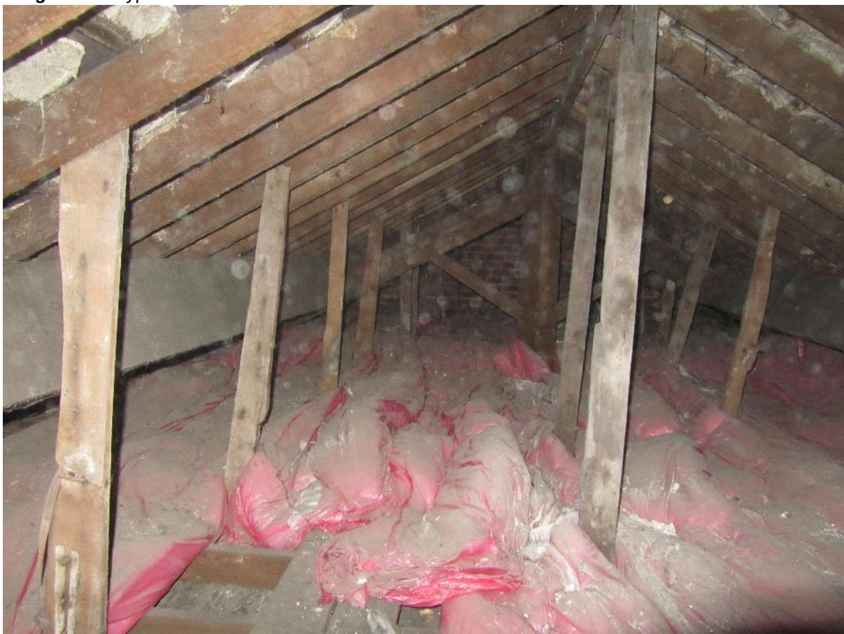
Image 3.19 A typical view within a loft void inside B1
