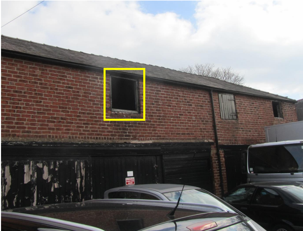
Image 3.33 Open window on the northern elevation of B3, from which a BLE emerged (indicated)
