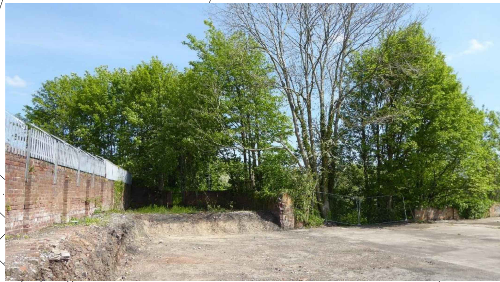
Photo looking towards north of site
