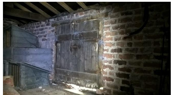
PHOTO 5.1 & 5.2. GAPS AT EAVES AND AROUND BOARDING
