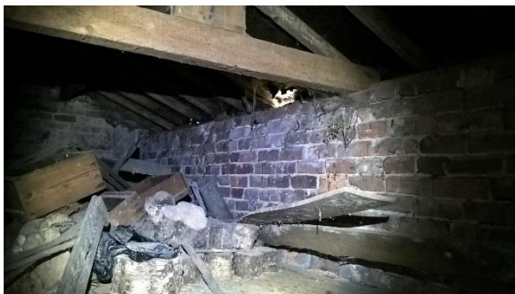
PHOTO 5.1 & 5.2. GAPS AT EAVES AND AROUND BOARDING
