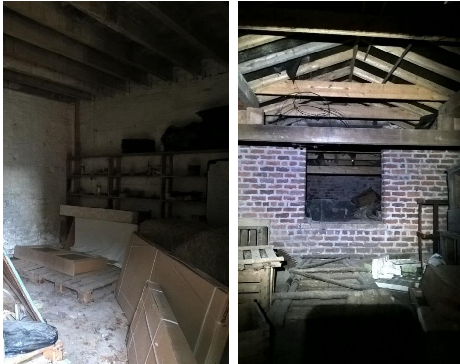
PHOTO 4.5 & 4.6. GROUND FLOOR AND FIRST FLOOR OF THE MAIN BUILDING.
