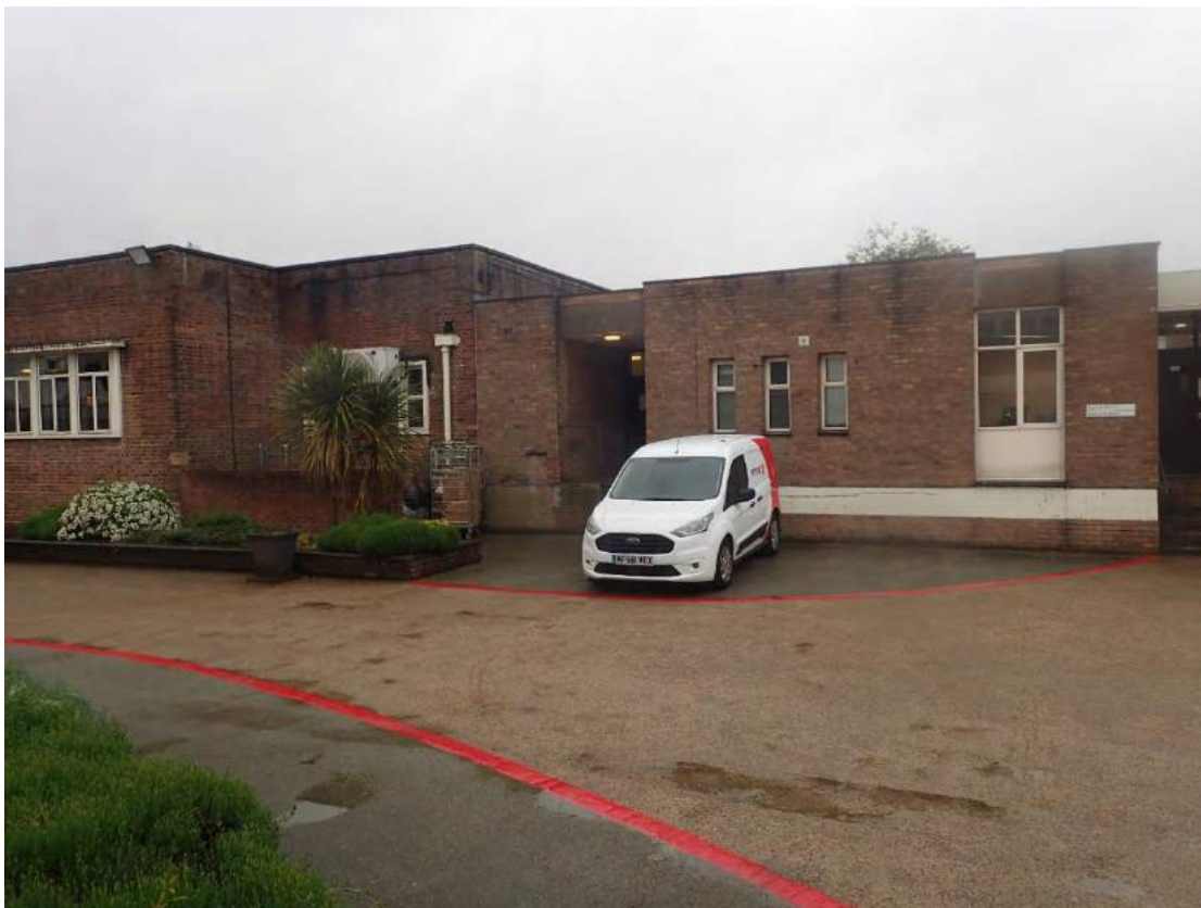
Image EDP 38: The north-east elevation of the 1960s extension to the Refectory at D-Block illustrating the join between the two buildings.
