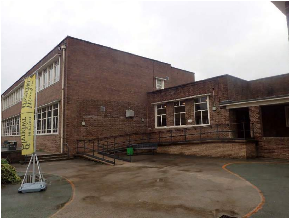
Image EDP 33: The side elevation of A-Block illustrating the second floor extension in the 1990s with the Refectory adjacent.
