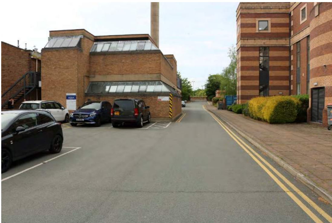
Image EDP 34: The construction department workshops to the north-west of the main part of the listed building.
