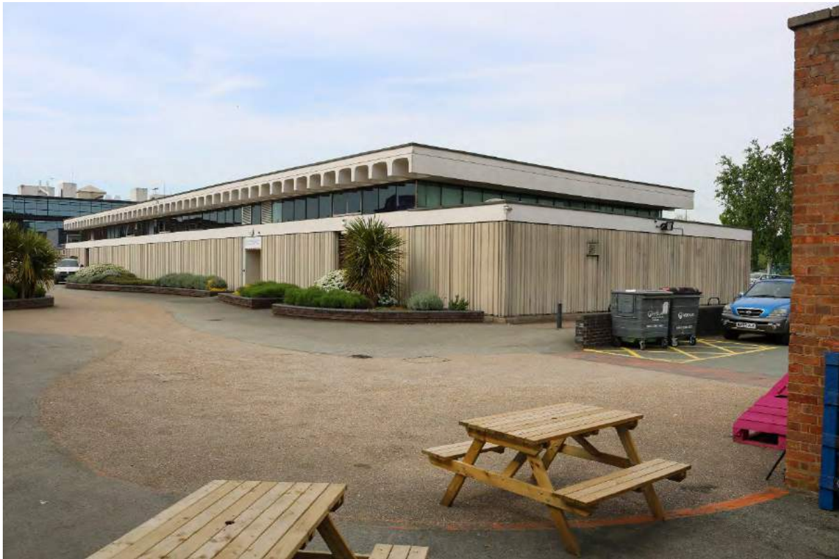
Image EDP 29: The later element of E-Block, viewed looking north-west and showing the characteristic form of construction.
