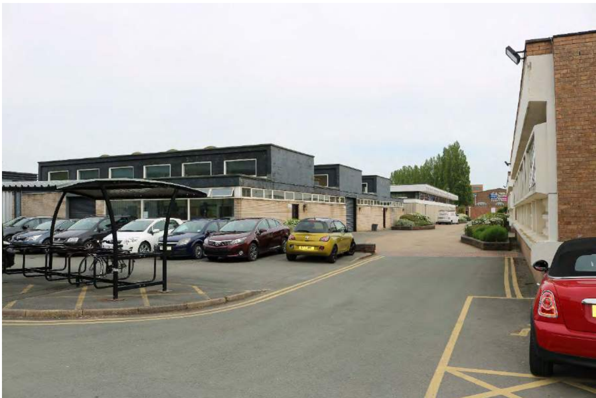
Image EDP 28: Typical view of E-Block (from the south-west) and illustrating the two separate structures and differing forms of construction.
