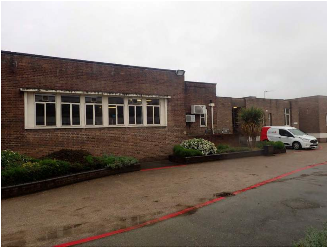
Image EDP 37: The north-east facing rear elevations of the Refectory.
