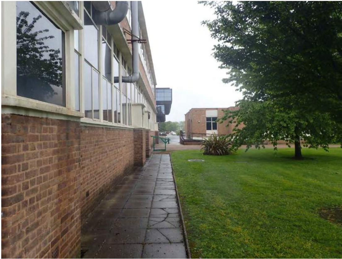
Image EDP 41: The building line between the listed building and the Edward Llwyd Centre viewed from the Quad.
