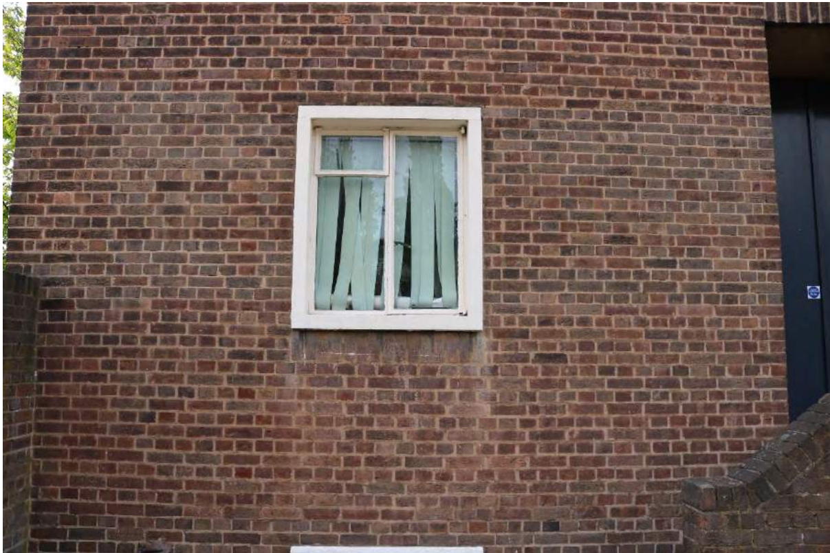
Image EDP 7: Close-up of an original window frame (one of just a few surviving examples).
