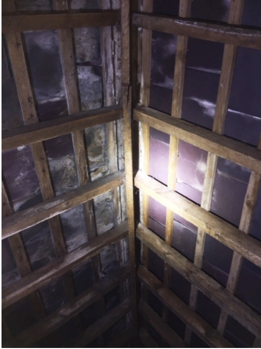
A1.5: Plate 5: Interior view of roof showing exposed wooden beams.
