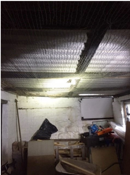
A1.6: Plate 6: Interior view of adjoining single storey garage of building.
