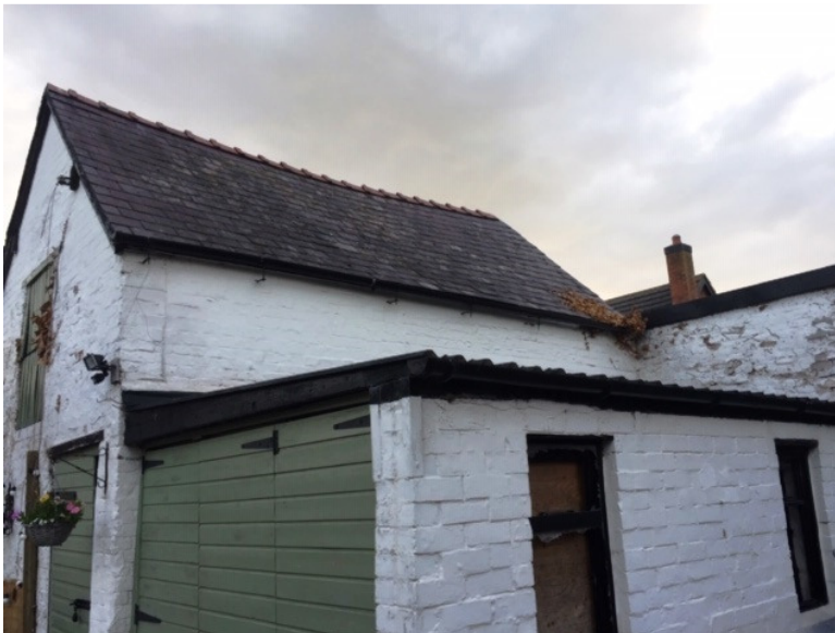
A1.2. Plate 2: View of the western side of building with adjoining single storey garage
