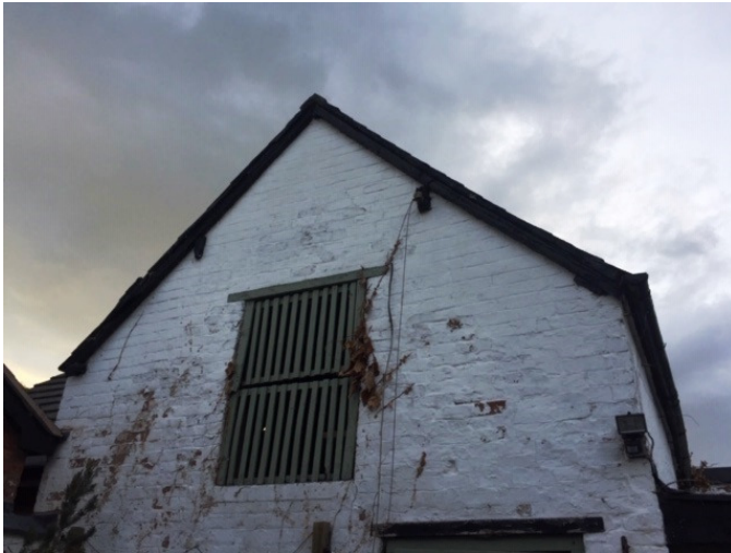
A1.1 Plate 1: View of the Southern Aspect of the building
