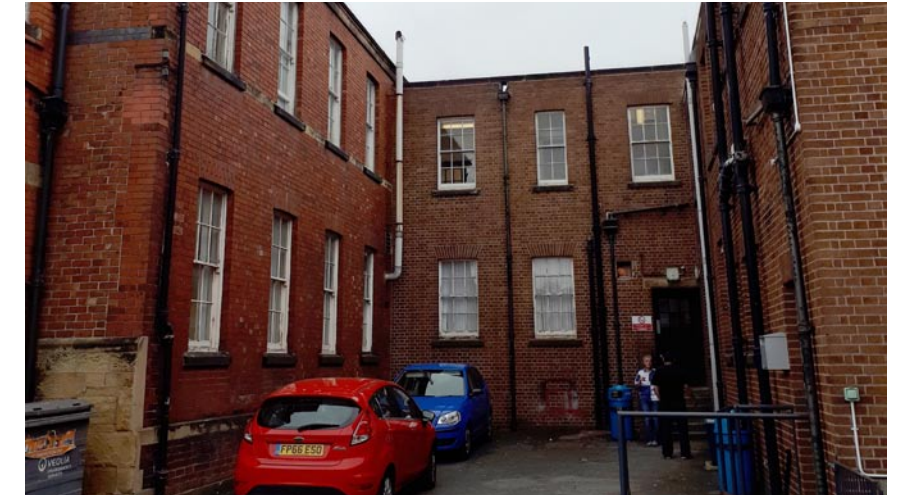
2. View of the existing courtyard
