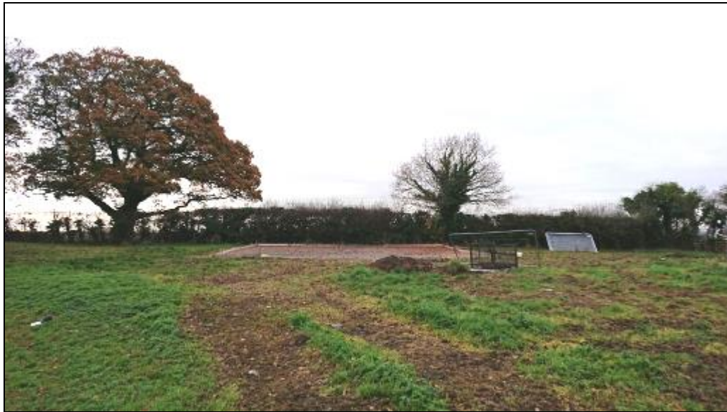
Plate 10 - Newly built building foundation, Target Note 5
