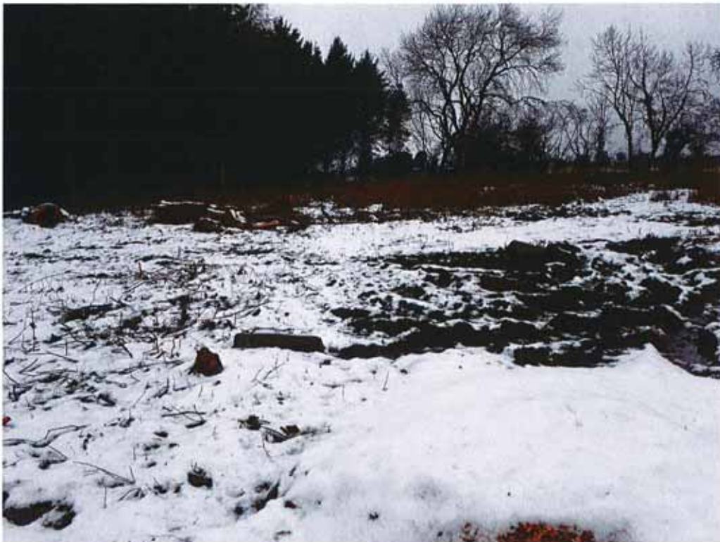
Photograph 3 – Northern part of the site following clearance works
