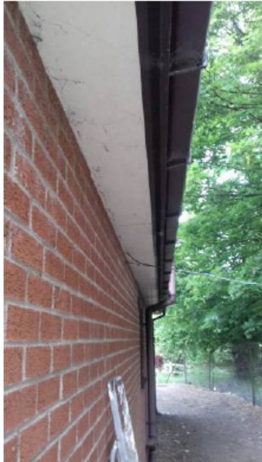
Side elevation soffits- close fitting to walls
