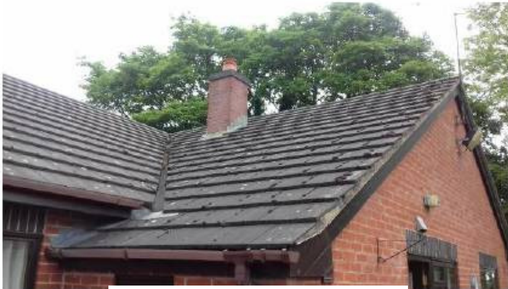
Roof & ridge tiles-close fitting
