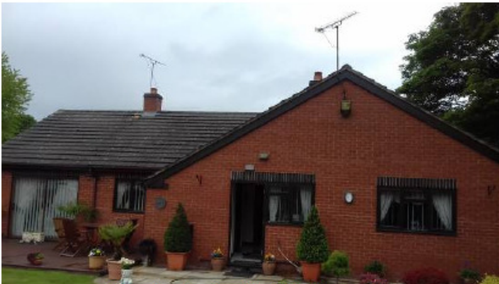
Rear elevation of residential property
