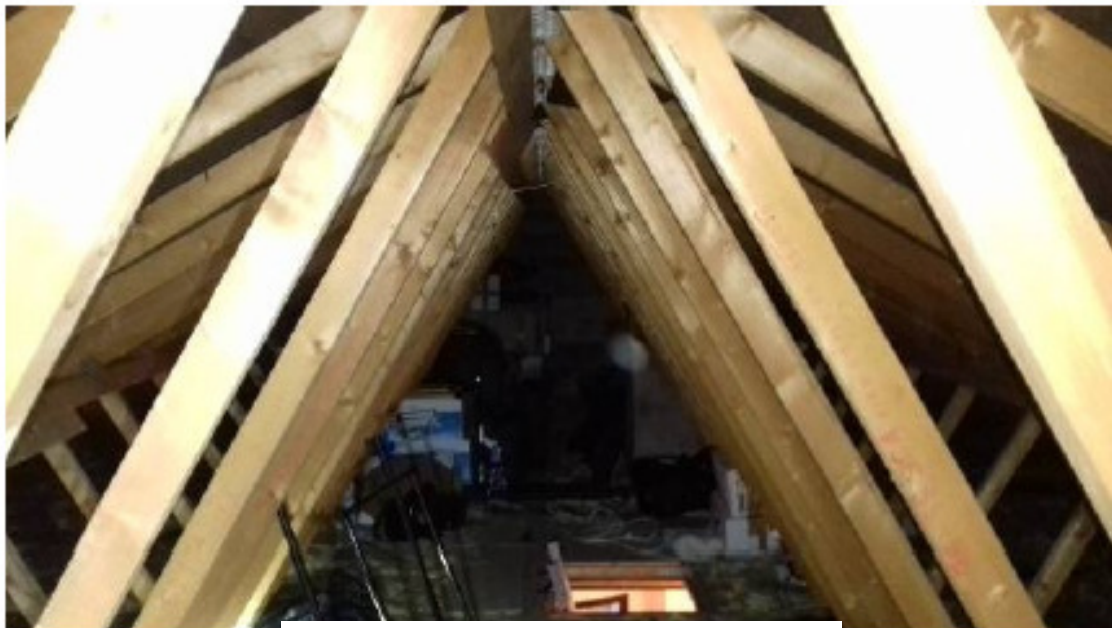
Restrictive truss roof design
