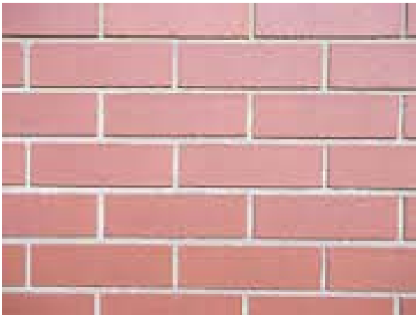
Red Engineering brick below DPC
