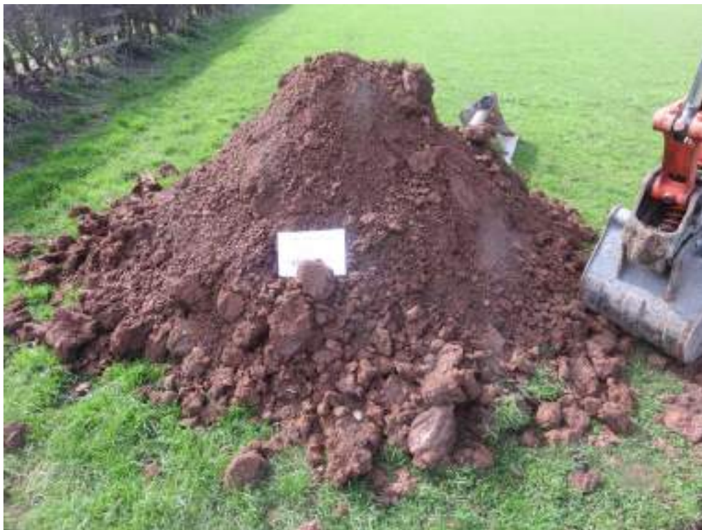
Photo 42 – Arising's from Trial Pit 21
