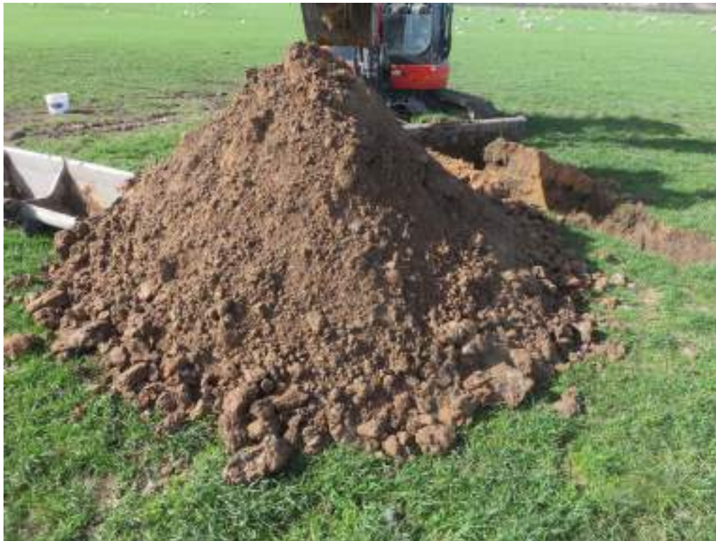
Photo 44 – Arising's from Trial Pit 22
