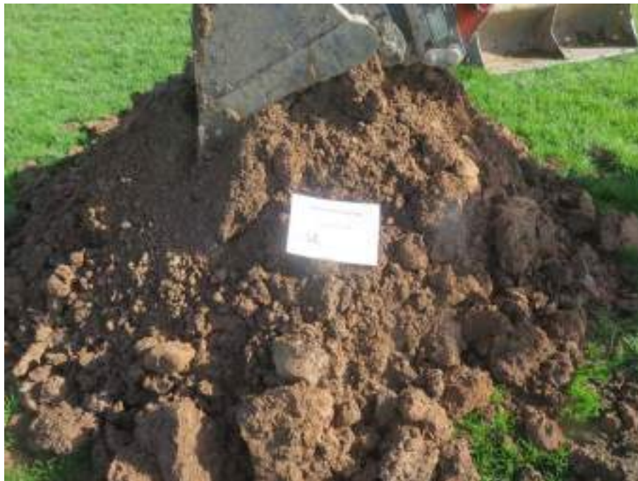
Photo 86 – Arising's from Trial Pit 42
