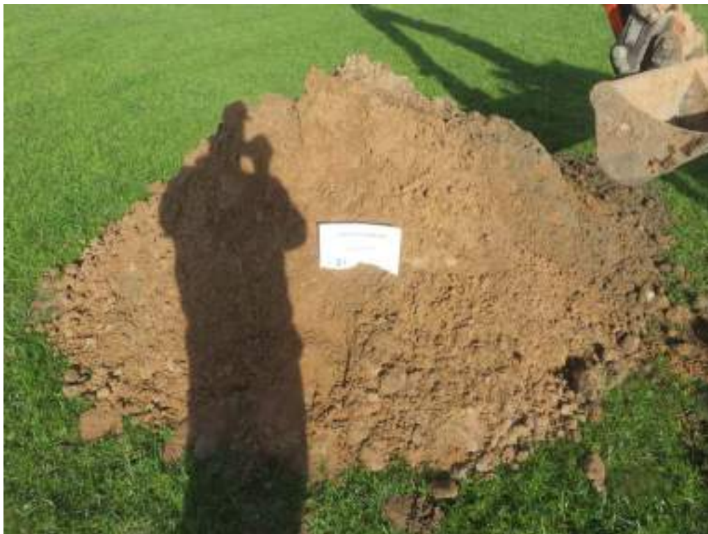
Photo 56 – Arising's from Trial Pit 28
