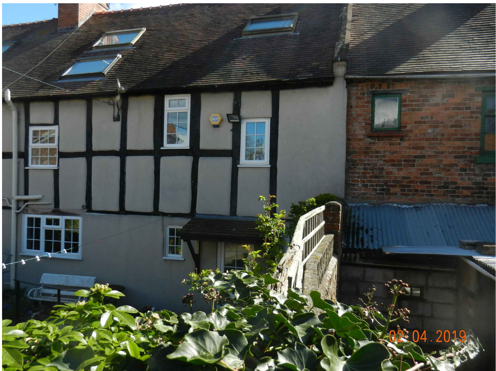
PHOTOGRAPH ALONG BOUNDARY
