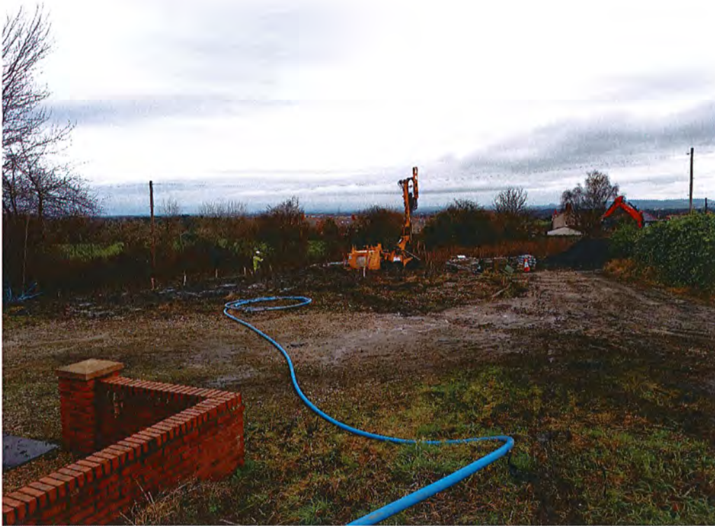
Photograph 3 Showing Plots 1 to 3
