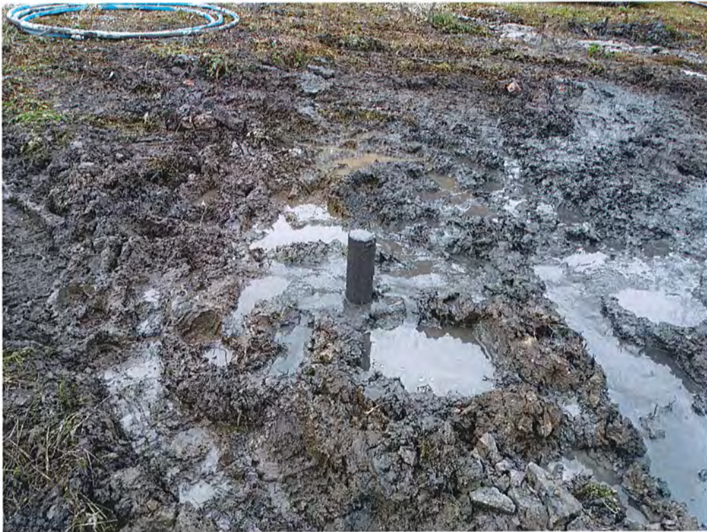
Photograph 1 Showing grout tremied to top of casing
