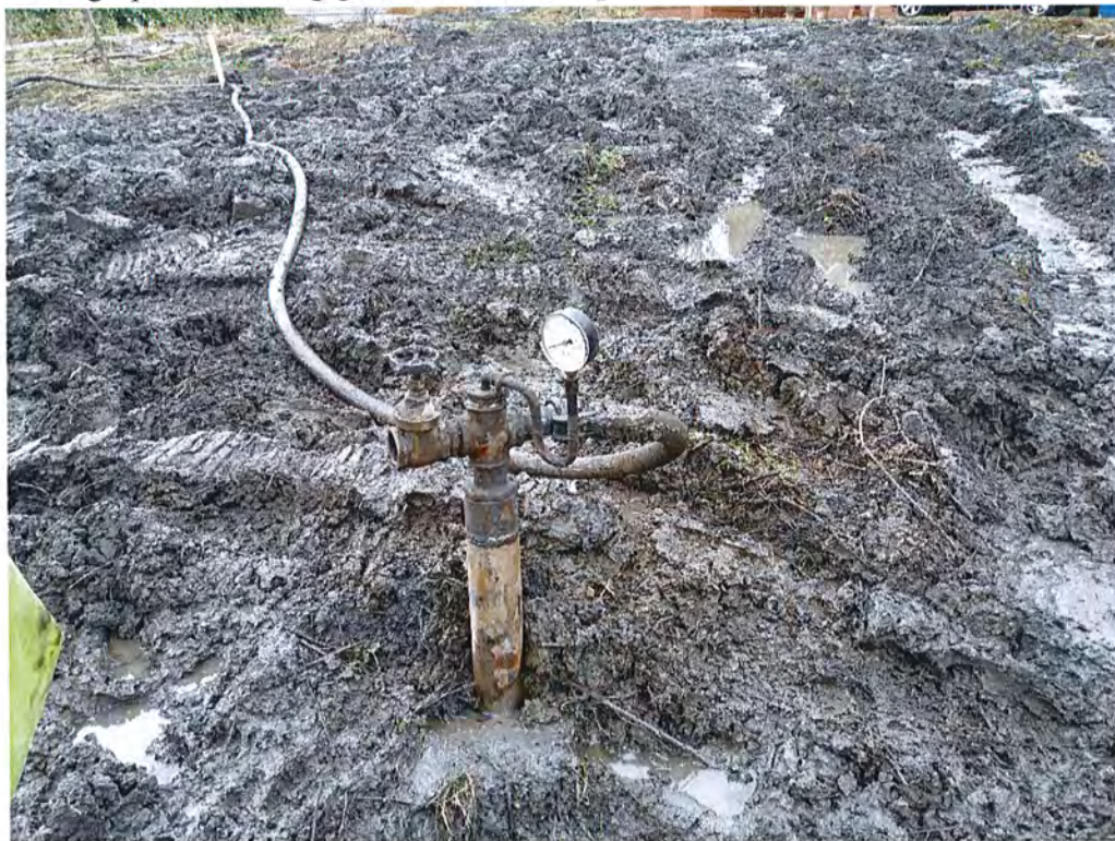
Photograph 2 Banjo attachment pressurising grout.
