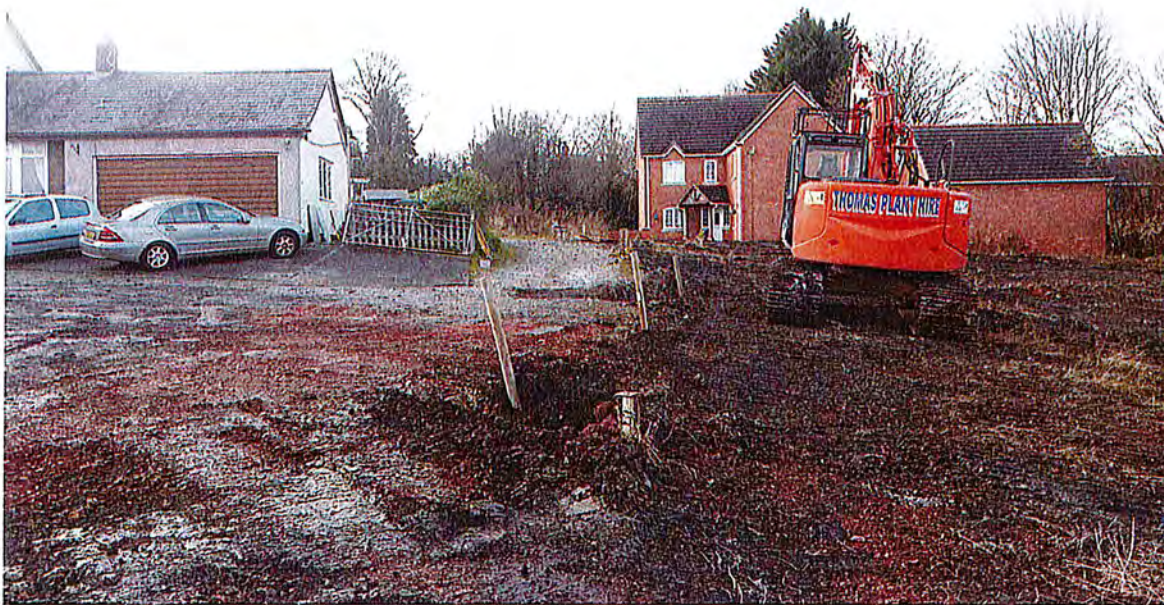
Photograph 5 Line of gas and water main looking west (posts)
