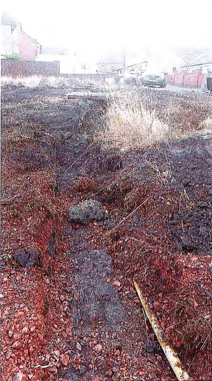
Photograph 12 Line of gas main
