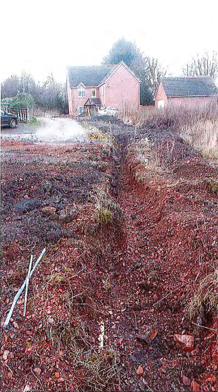
Photograph 11 Line of gas main
